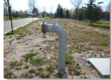
Figure 1: Drafting Port Side View - 90 Deg Elbow
