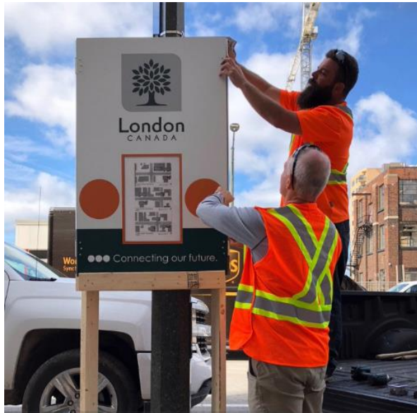
Core construction notice sign installation outside of downtown apartment building.
