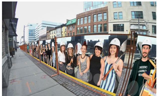
Dundas Place construction barrier signage featuring community members
