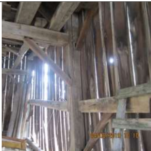
Image 35. Interior of Barn 2 located at 3303 Westdel Bourne. April 2019.
