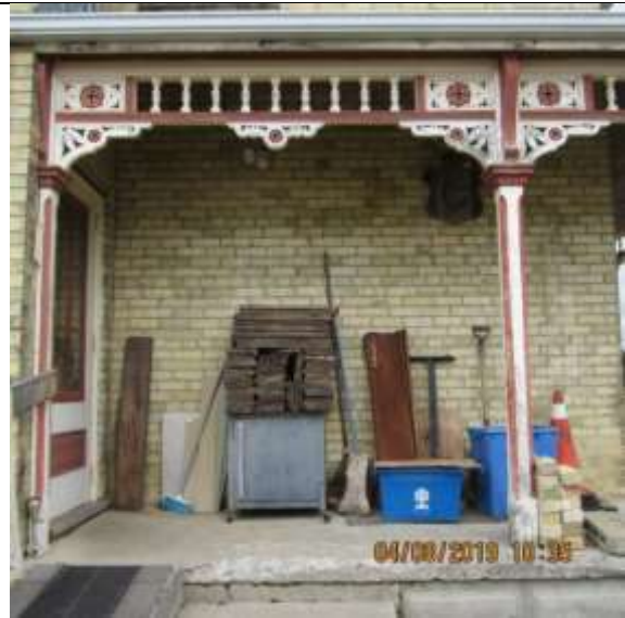
Image 19. Front façade of the farmhouse located at 3303 Westdel Bourne, looking west. April 2019.
