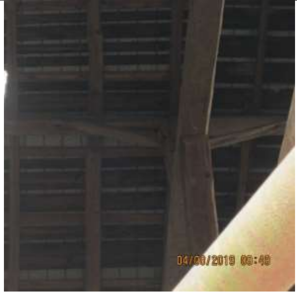
Image 31. Interior of Barn 1 located at 3303 Westdel Bourne. April 2019.
