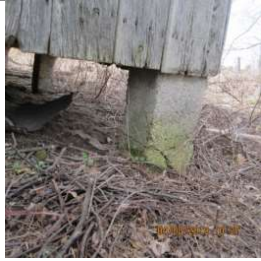
Image 37. Close up of concrete pillars. Barn 3 located at 3303 Westdel Bourne. April 2019.
