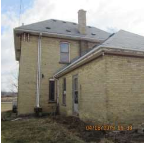
Image 6. Rear façade of the farmhouse located at 3303 Westdel Bourne. April 2019.
