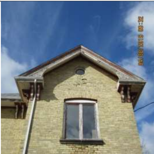
Image 10. Front façade of the farmhouse located at 3303 Westdel Bourne. April 2019.
