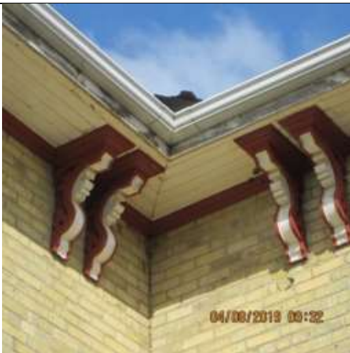
Image 14. Example of the paired brackets at the farmhouse located at 3303 Westdel Bourne. April 2019.
