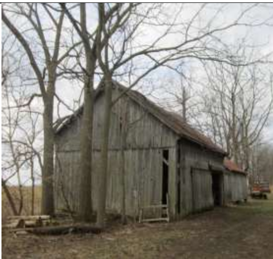
Image 34. East façade of Barn 2 located at 3303 Westdel Bourne. April 2019.
