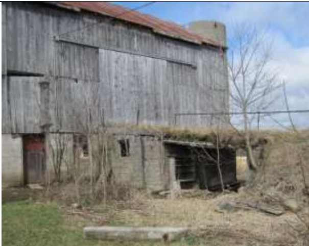
Image 32. Photo of the Barn Hill. Barn 1 located at 3303 Westdel Bourne. April 2019.
