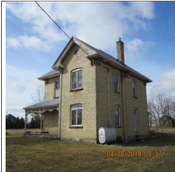
Image 4. Front and north façade of the farmhouse located at 3303 Westdel Bourne. April 2019.
