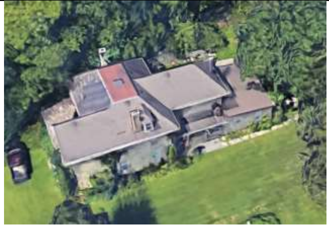
Image 39 – 2420 Westdel Bourne, c. 1875. East façade. Property not able to be seen from the street. Heritage listed property. Photo courtesy of Google Streetview.
