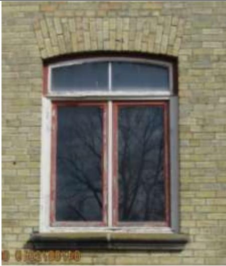
Image 12. Window example, front façade of the farmhouse located at 3303 Westdel Bourne. April 2019.
