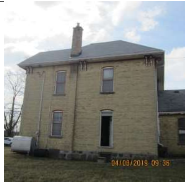
Image 5. North façade of the farmhouse located at 3303 Westdel Bourne. April 2019.
