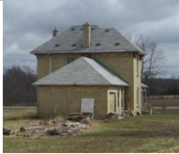
Image 7. Rear façade of the farmhouse located at 3303 Westdel Bourne. April 2019.
