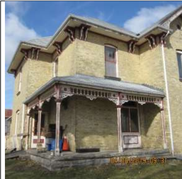
Image 18. Front façade of the farmhouse located at 3303 Westdel Bourne. April 2019.
