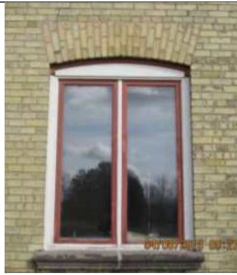
Image 11 Window example, front façade of the farmhouse located at 3303 Westdel Bourne. April 2019.
