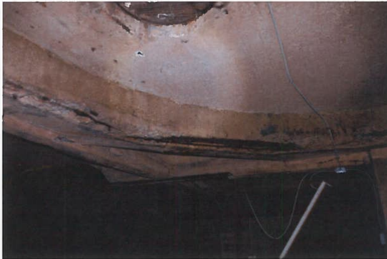
Photo No 09: Interior Basement Beams (south end)
