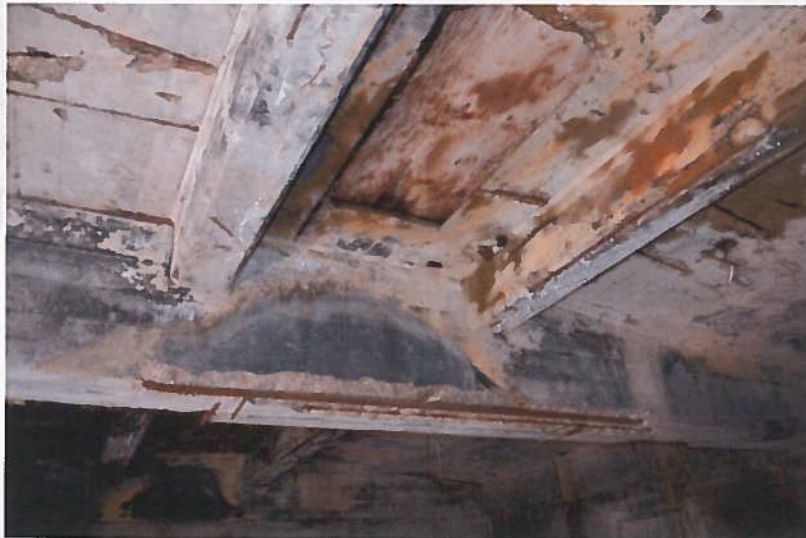
Photo No 08: Typical Interior Upper Beam
