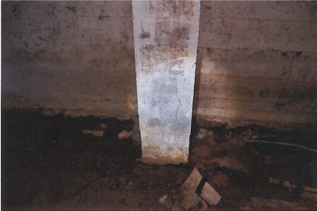
Photo No 03: Concrete Foundation Walls
