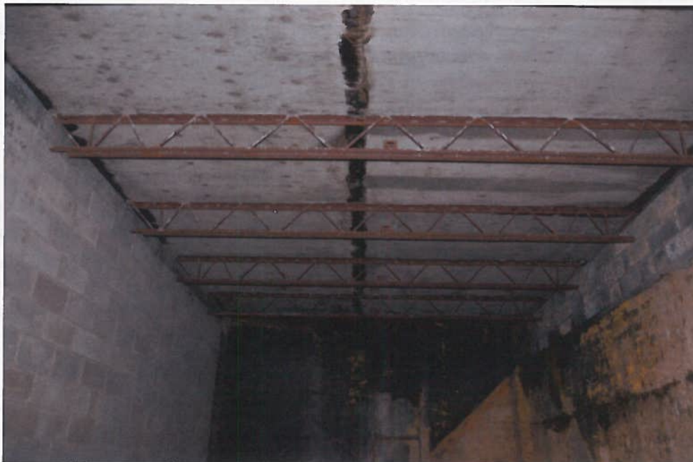
Photo No 02: Added Hambro Floor System
