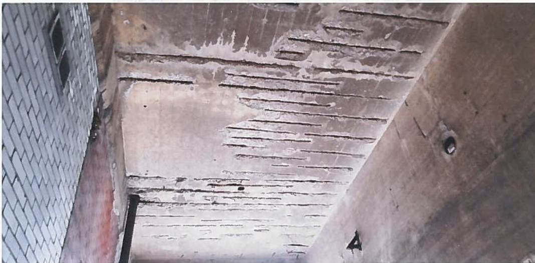
Photo No 06: Suspended Link Slab (Exterior)
