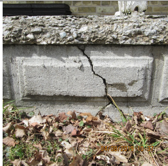
Image 25. Close of up of the concrete base of the verandah. Front façade of the farmhouse located at 3303 Westdel Bourne. April 2019.
