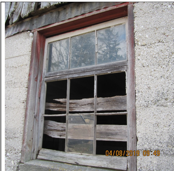
Image 28. Window example. Barn 1 located at 3303 Westdel Bourne. April 2019.
