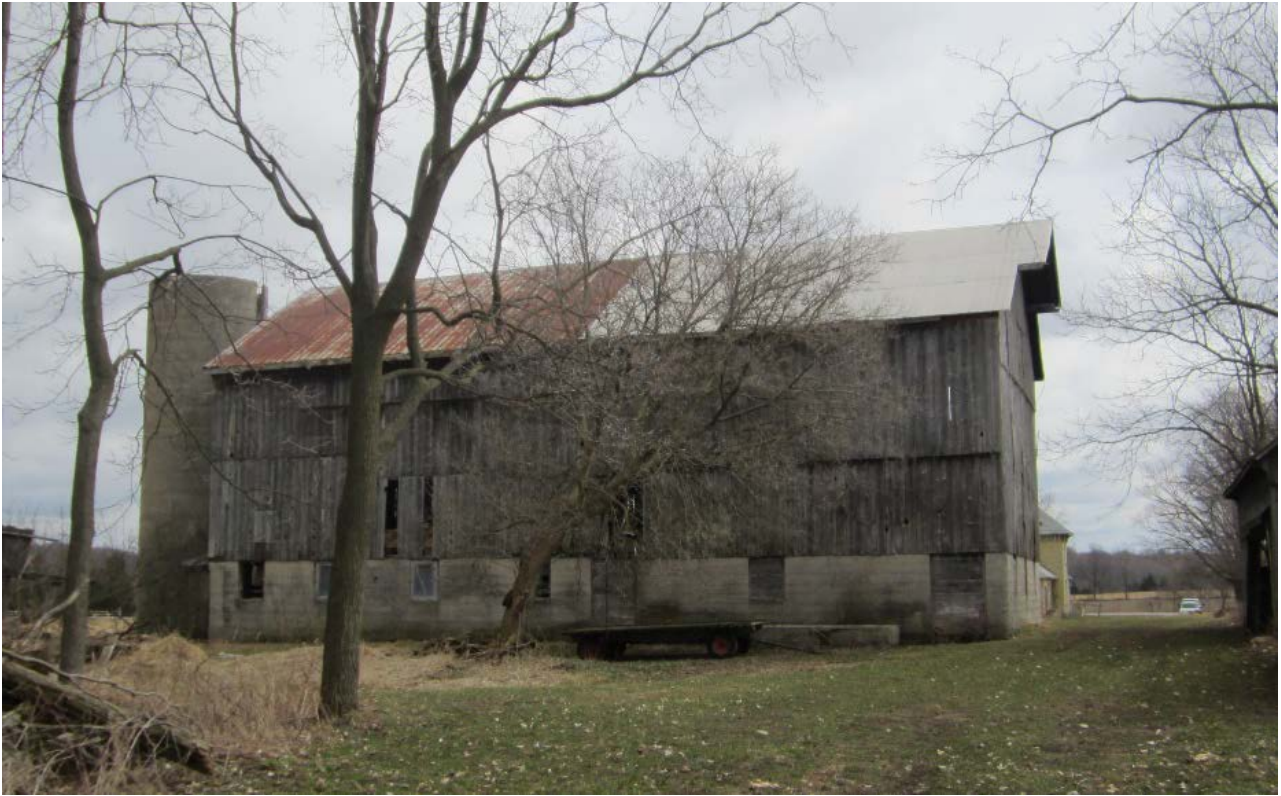
Image 27. West façade of Barn 1 located at 3303 Westdel Bourne, looking east. April 2019.
