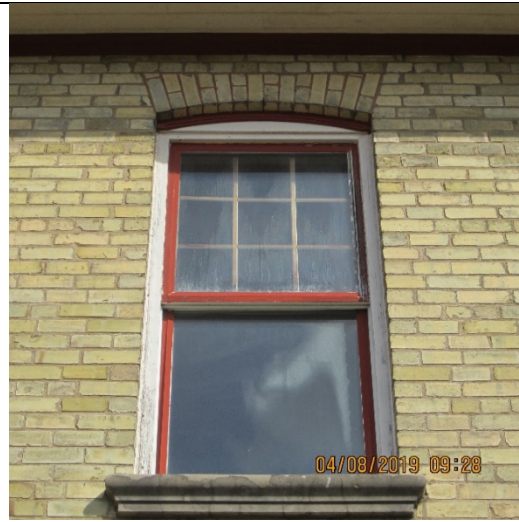
Image 13. Window example, south façade of the farmhouse located at 3303 Westdel Bourne, looking west. April 2019.
