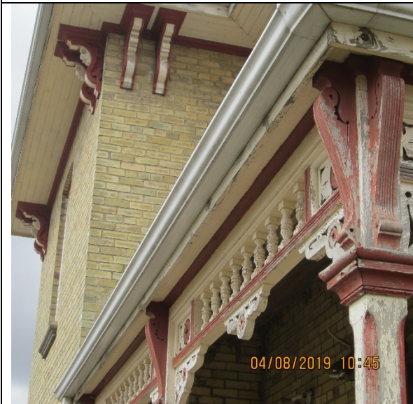
Image 20. Close up of verandah detail. Front façade of the farmhouse located at 3303 Westdel Bourne. April 2019.
