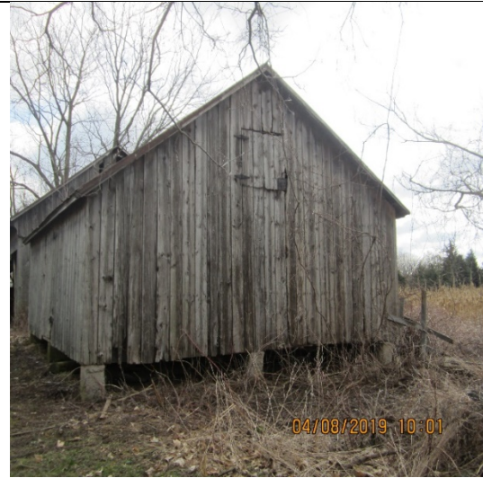
Image 36. West façade of Barn 3 located at 3303 Westdel Bourne. April 2019.
