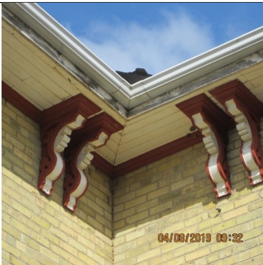
Image 14. Example of the paired brackets at the farmhouse located at 3303 Westdel Bourne. April 2019.
