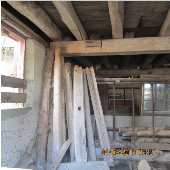
Image 30. Interior of Barn 1 located at 3303 Westdel Bourne. April 2019.
