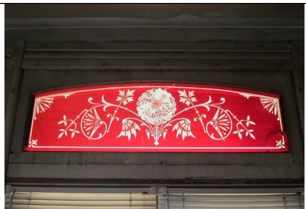
Image 17. Etched glass above original front door opening. Interior photo of the farmhouse located at 3303 Westdel Bourne. April 2019.
