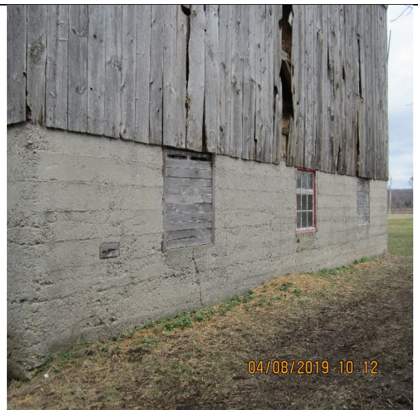
Image 29. Parged concrete foundation. Barn 1 located at 3303 Westdel Bourne. April 2019.
