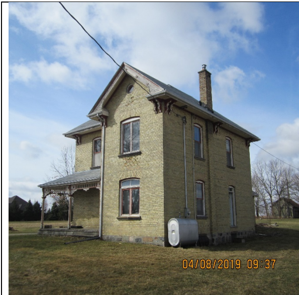
Image 4. Front and north façade of the farmhouse located at 3303 Westdel Bourne. April 2019.
