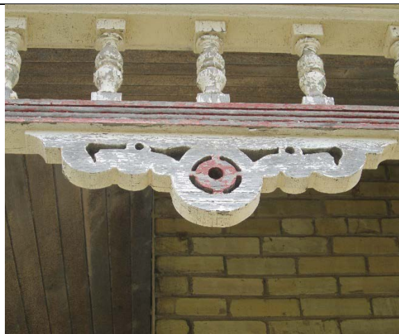
Image 23. Close up of verandah details. Front façade of the farmhouse located at 3303 Westdel Bourne. April 2019.
