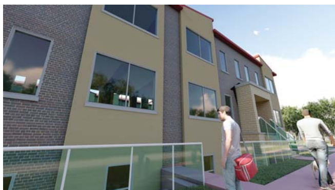
Public sidewalk at the front and its proximity to the building
