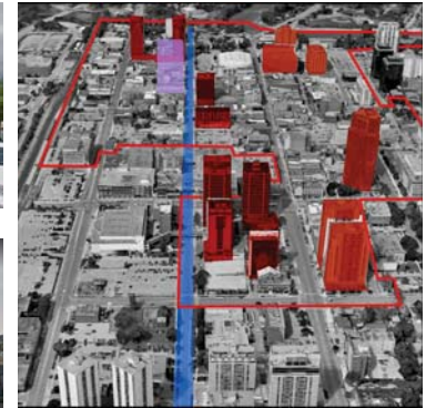
Aerial photograph of Downtown HCD highlighting multi-storey buildings. King St. is shaded blue, 131 King shaded violet
