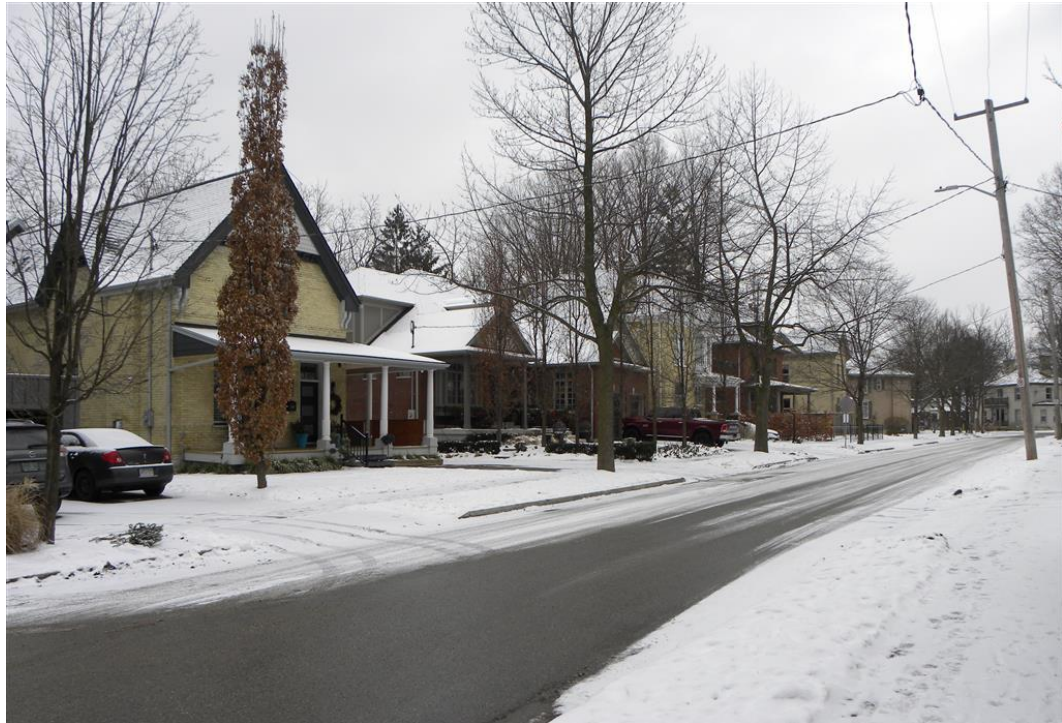
Figure 12: Streetscape facing west on The Ridgeway (January 18, 2019).
