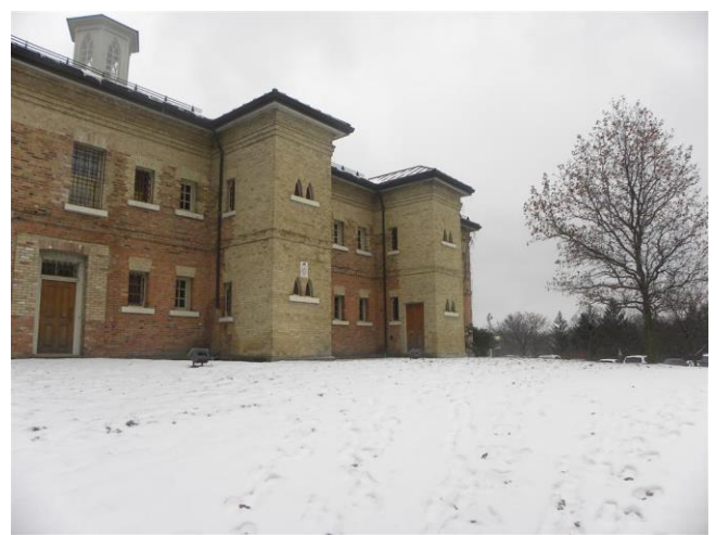
West façade of the Gaol (January 18, 2019)
