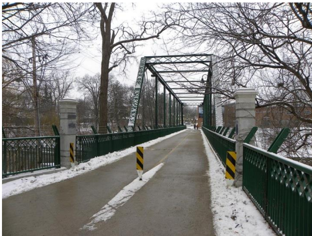
View west across King Street Bridge (January 18, 2019)
