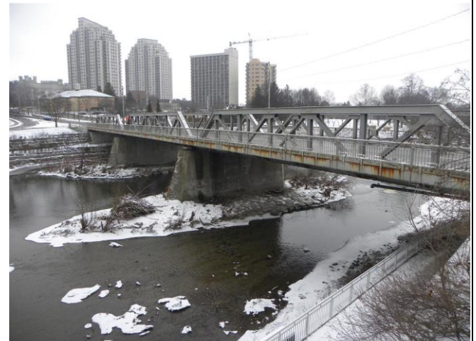
North side of Kensington Bridge (January 18, 2019)
