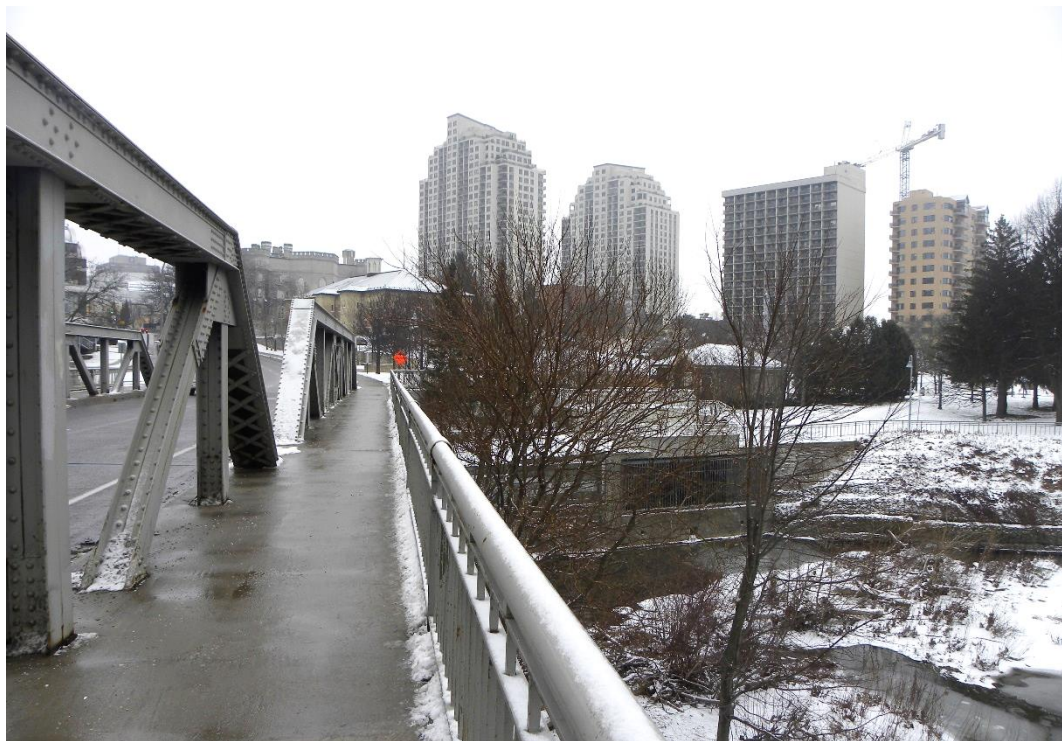
Figure 27: Kensington Bridge facing east (January 18, 2019).
