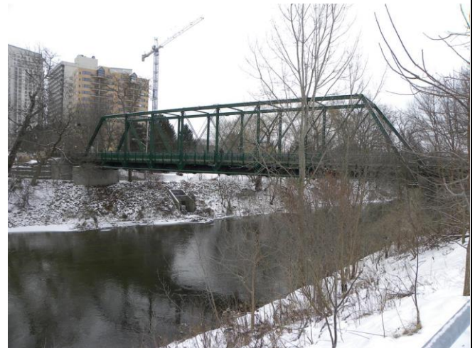
North side of King Street Bridge (January 18, 2019)
