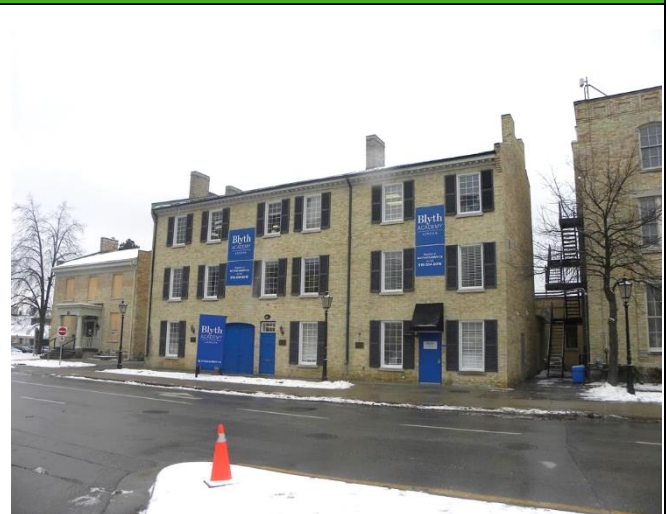
East façade, Gore Bank and Bank of Upper Canada (January 18, 2019)
