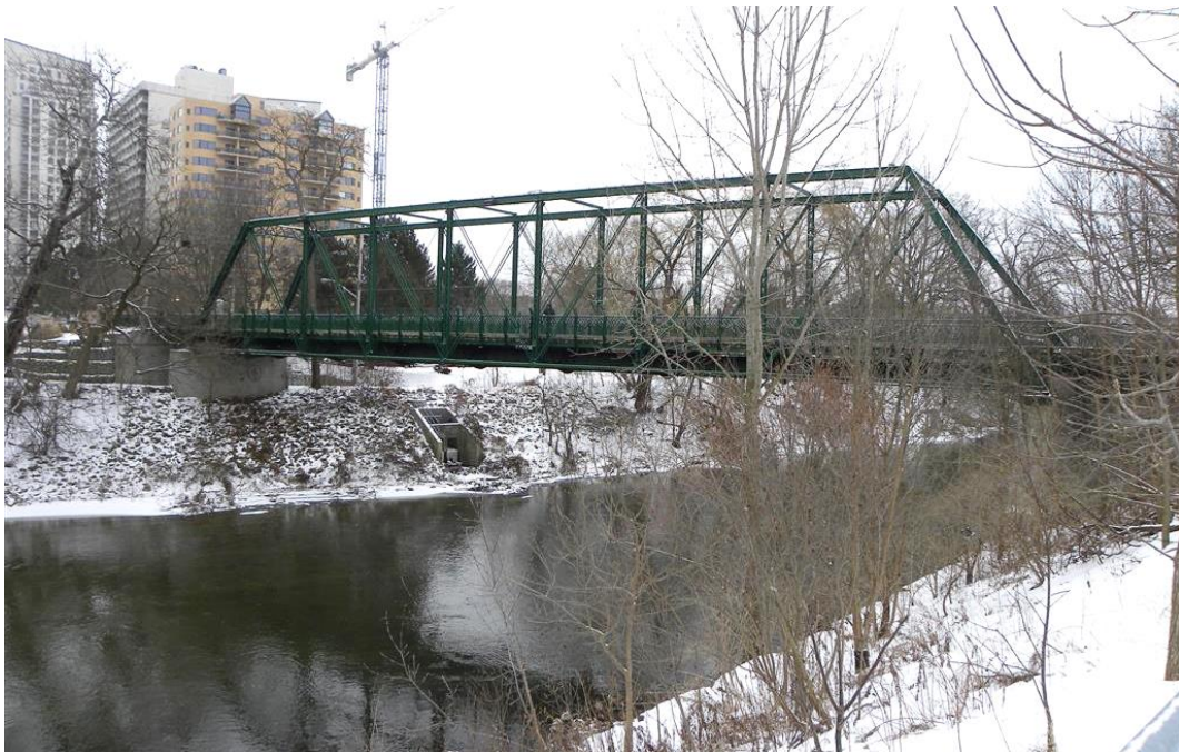
Figure 21: King Street Bridge, facing southeast (January 18, 2019).
