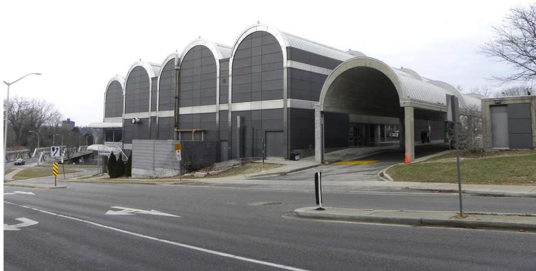
Figure 43: South and east facades of Museum London (421 Ridout Street North; March 28, 2019).
