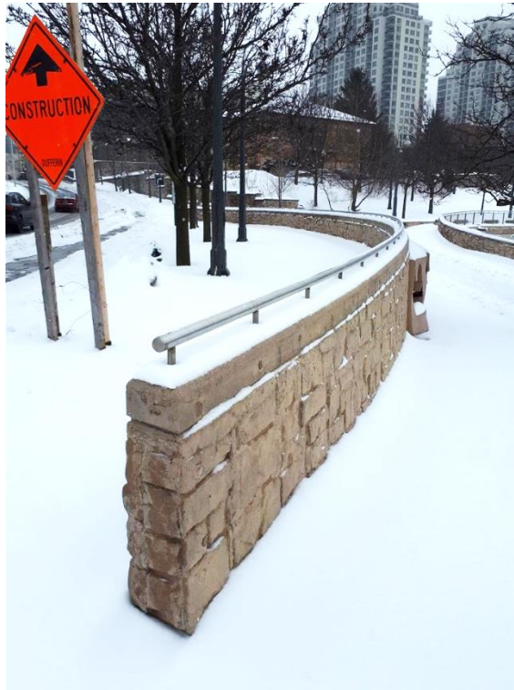
Figure 39: South end of the study area (Ivey Park), looking east with Gaol in background (January 29, 2019).
