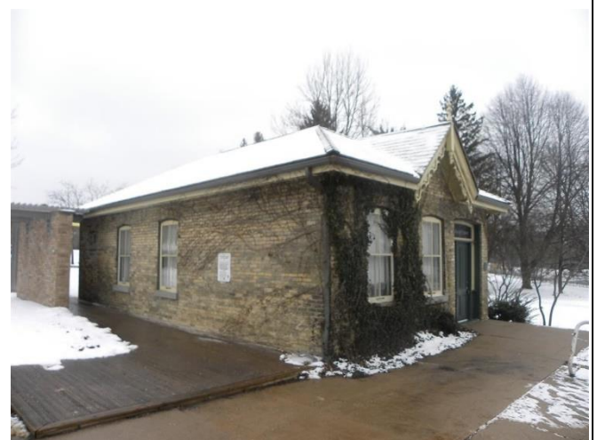
North and east façades (January 18, 2019)
