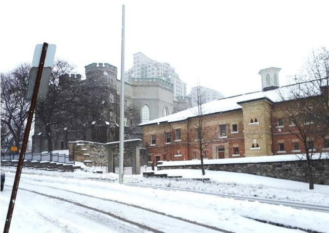
North and west facades of the Court House and Gaol (January 29, 2019)
