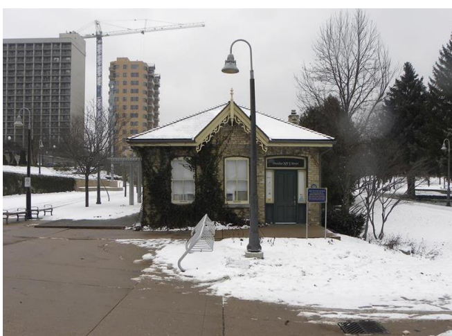
North façade (January 18, 2019)
