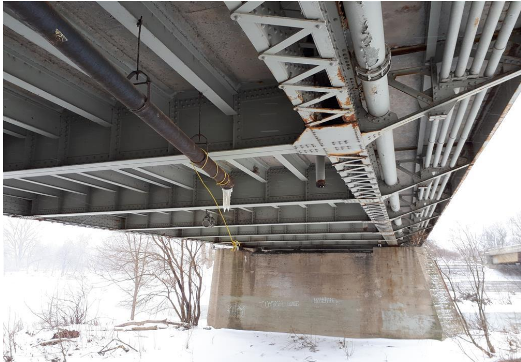
Figure 30: Underside of the Kensington Bridge, facing west (January 29, 2019).
