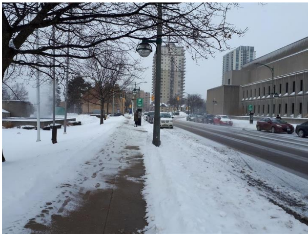
View north on Ridout Street North (January 29, 2019)
