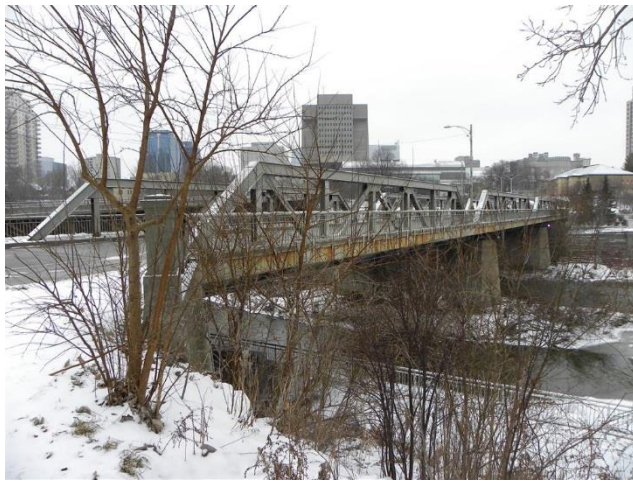
South side of Kensington Bridge (January 18, 2019)
