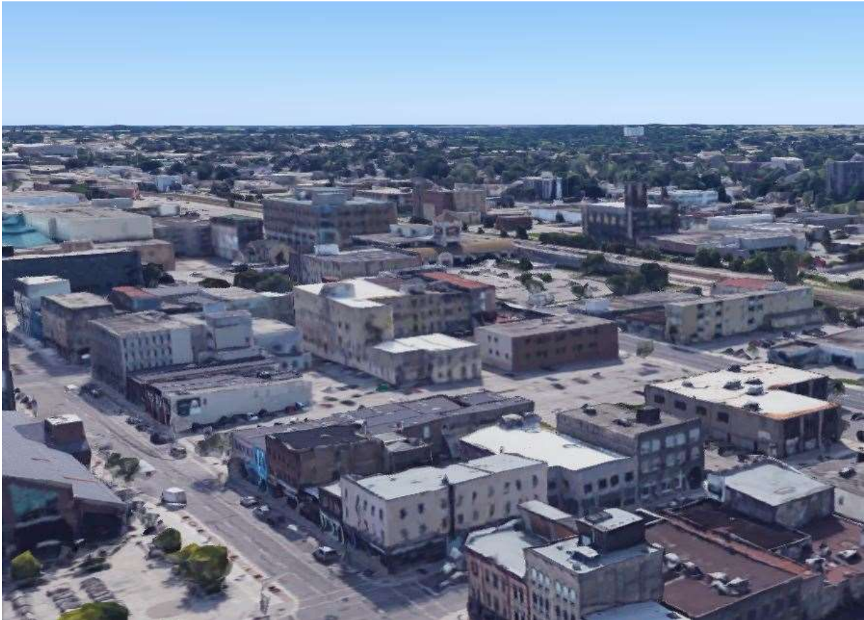
Image 2: Aerial view of block at the corner of King and Talbot Streets – facing south east
