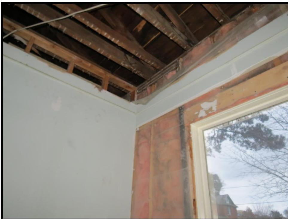
**Image 30: Detail of ceiling joists, wood trim and window surrounds in middle room (west)**
