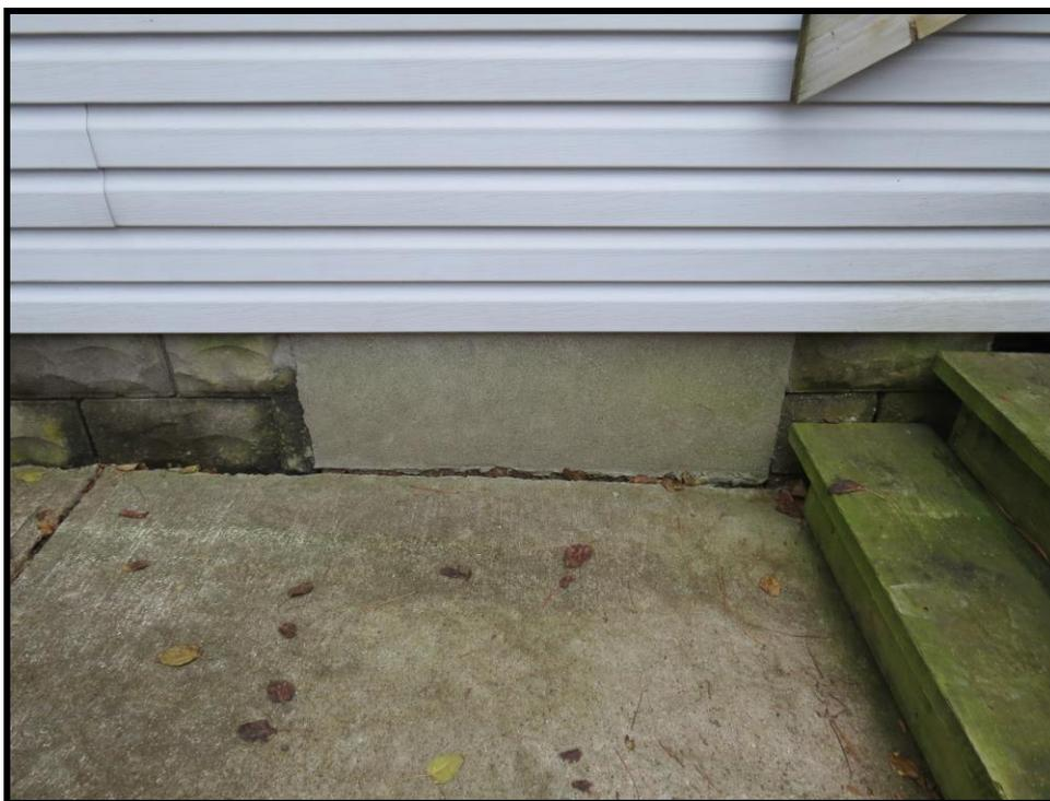
**Image 14: Detail of enclosed basement window opening on north elevation**
