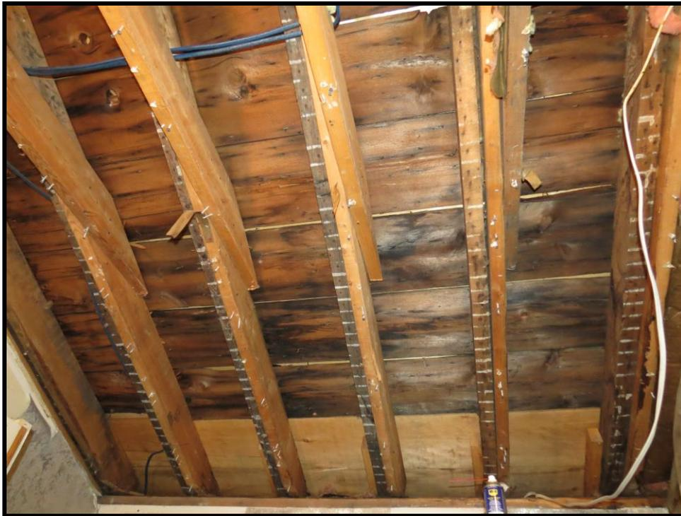
**Image 35: Detail of ceiling joists in rear addition**
