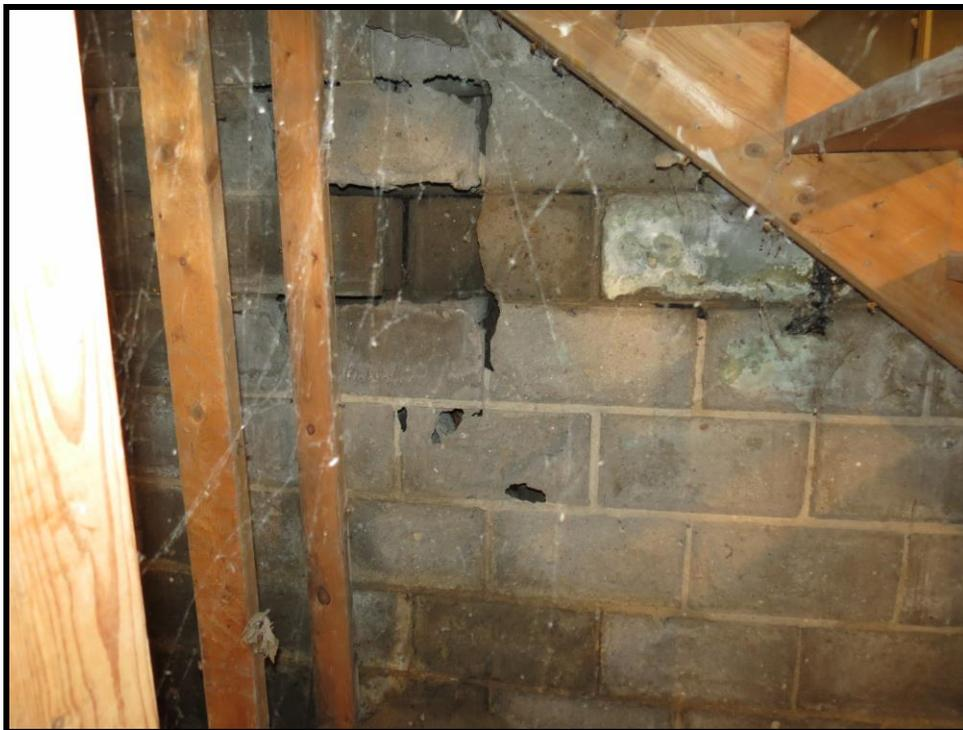
**Image 40: Detail of condition of cinderblock basement wall construction**
