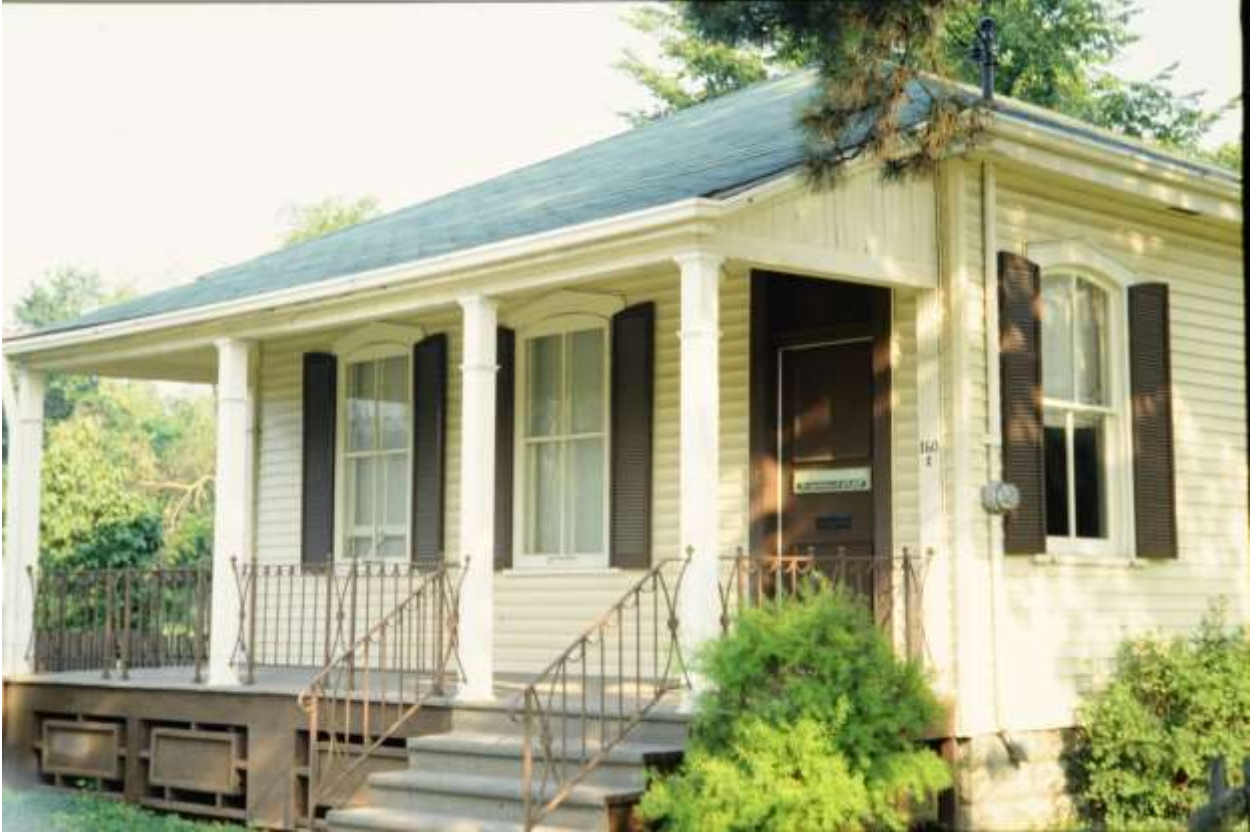
Image 1: Converted slide image of the subject property at 160 Oxford Street East (not dated). Noted the metal railing and porch skirting, as well as the hoods above the window openings with segmented-arch two-over-two wood windows (storm windows on front windows under verandah).
