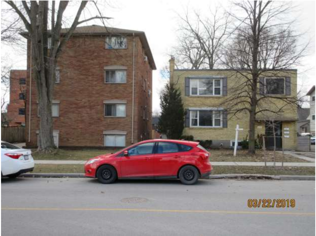
Image 8: Adjacent and nearby properties on St. George Street, north of the subject property.
