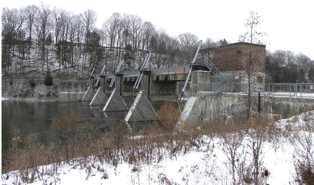
Figure 12: West side of the Springbank Dam, facing northeast (January 18, 2019).
