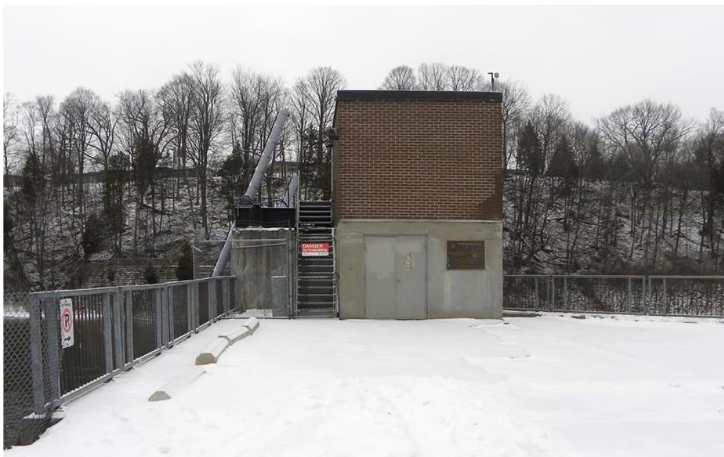
Figure 13: South side of the Springbank Dam, facing north (January 18, 2019).
