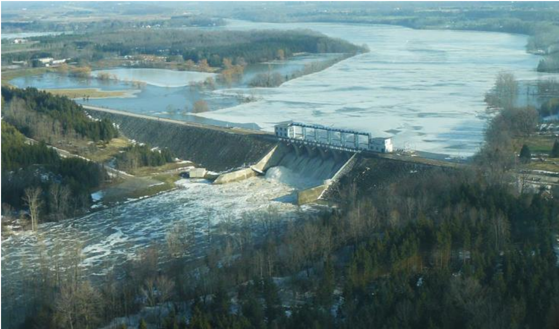
Figure 19: Fanshawe Dam, 2008 (UTRCA 2019).
