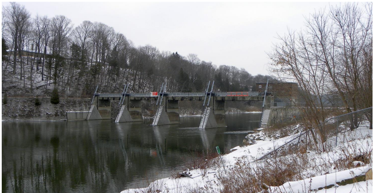
Figure 11: West side of the Springbank Dam, facing east (January 18, 2019).
