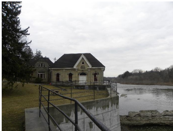
View facing west of the Pumphouse and remnants of the dam (March 28, 2019)
