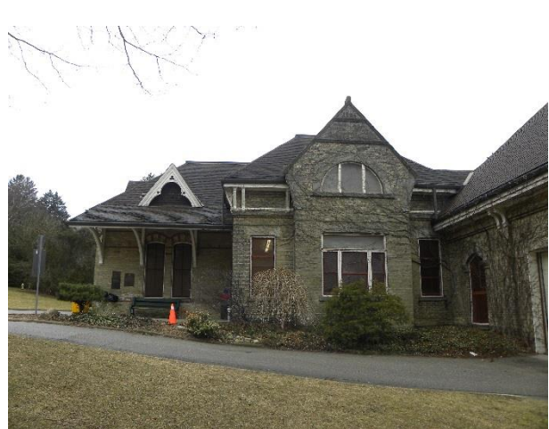
South portion of the Pumphouse (March 28, 2019)
