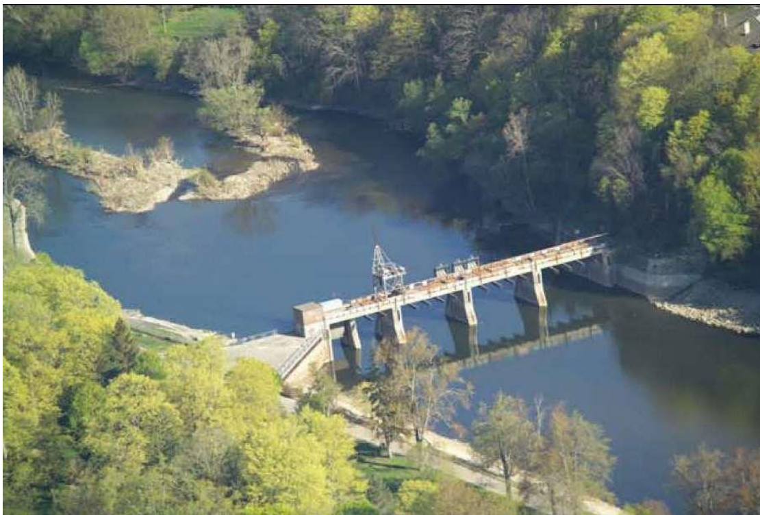
Figure 9: Aerial view of the Springbank Dam, pre-2006 (One River Stage 2 2018:9).
