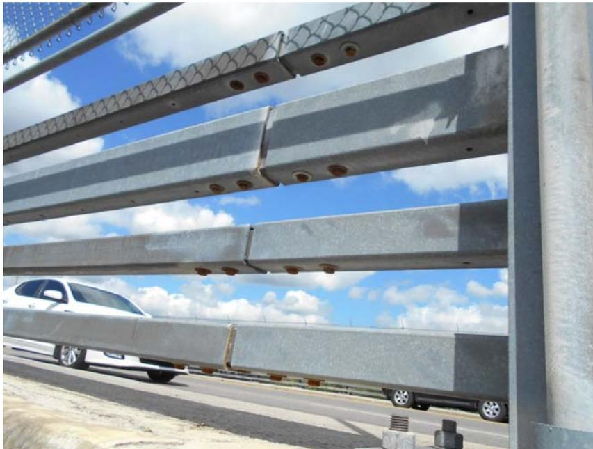
***CORROSION ON THE RAILING-AUG'15***
