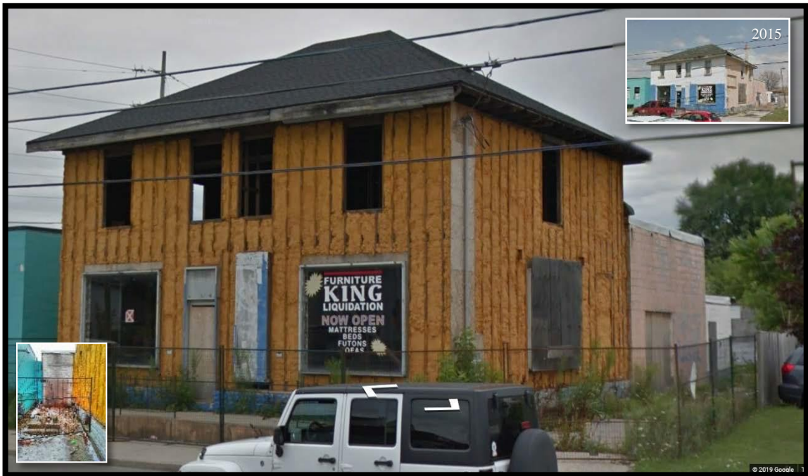
Photo of Subject Property – 200 Adelaide Street North – Exterior Condition
