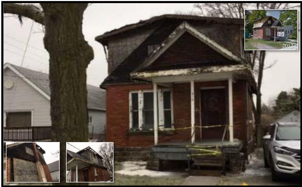
Photo of Subject Property – 315 Oakland Avenue – Exterior Condition
