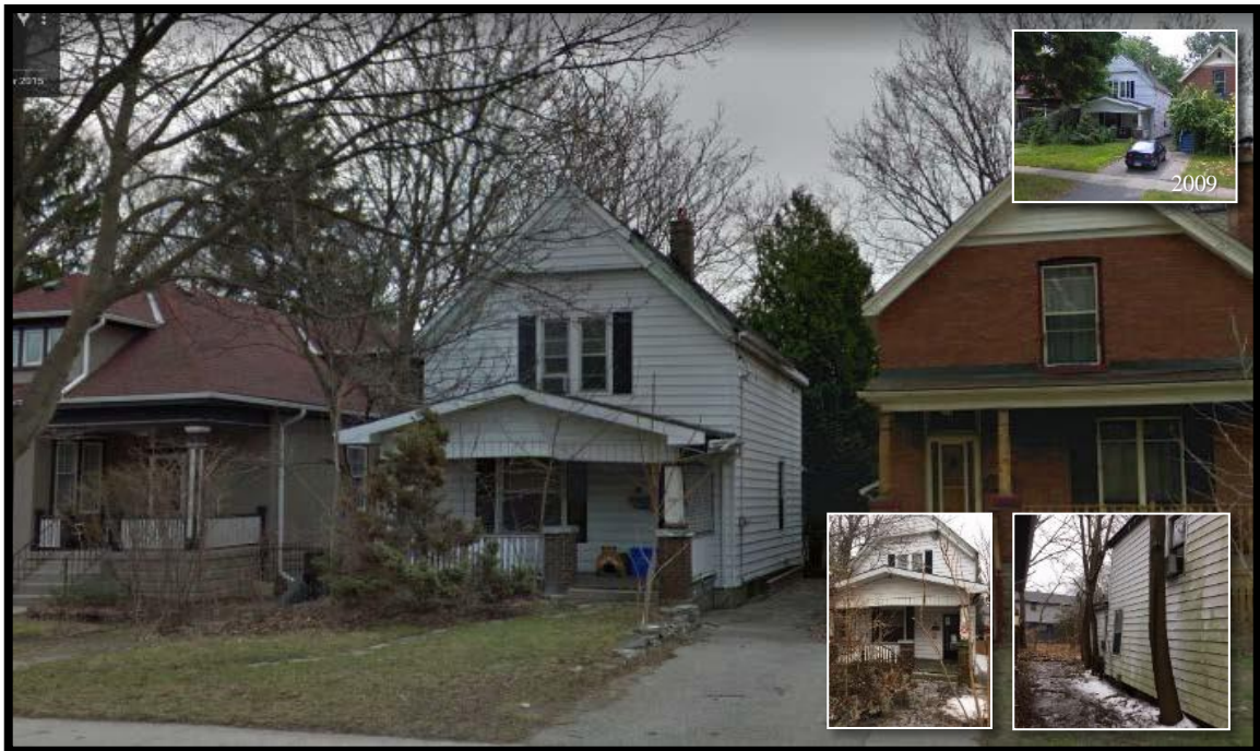
Photo of Subject Property – 533 Piccadilly Street – Exterior Condition
