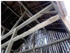
View of barn interior illustrating exterior bent, west face
