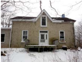
Front façade of farmhouse – north face, facing Kilally Road
