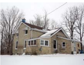
Side elevation of house – west-south corner, with additions to original farmhouse
