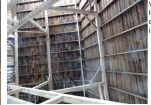
View looking up of barn interior
