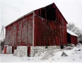
View of barn, east-south corner illustrating gangway, rubble foundation and lower stable level
