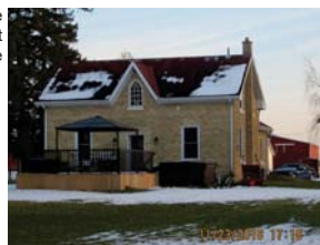
1511 Clarke Road, front façade
