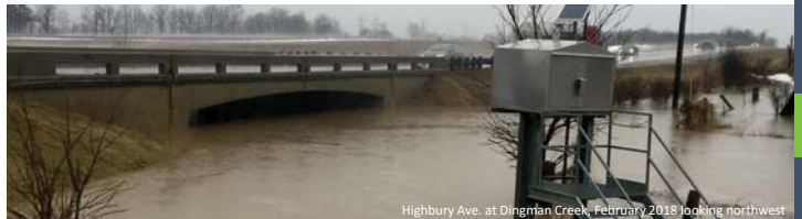
Highbury Ave. at Dingman Creek, February 2018 looking northwest
