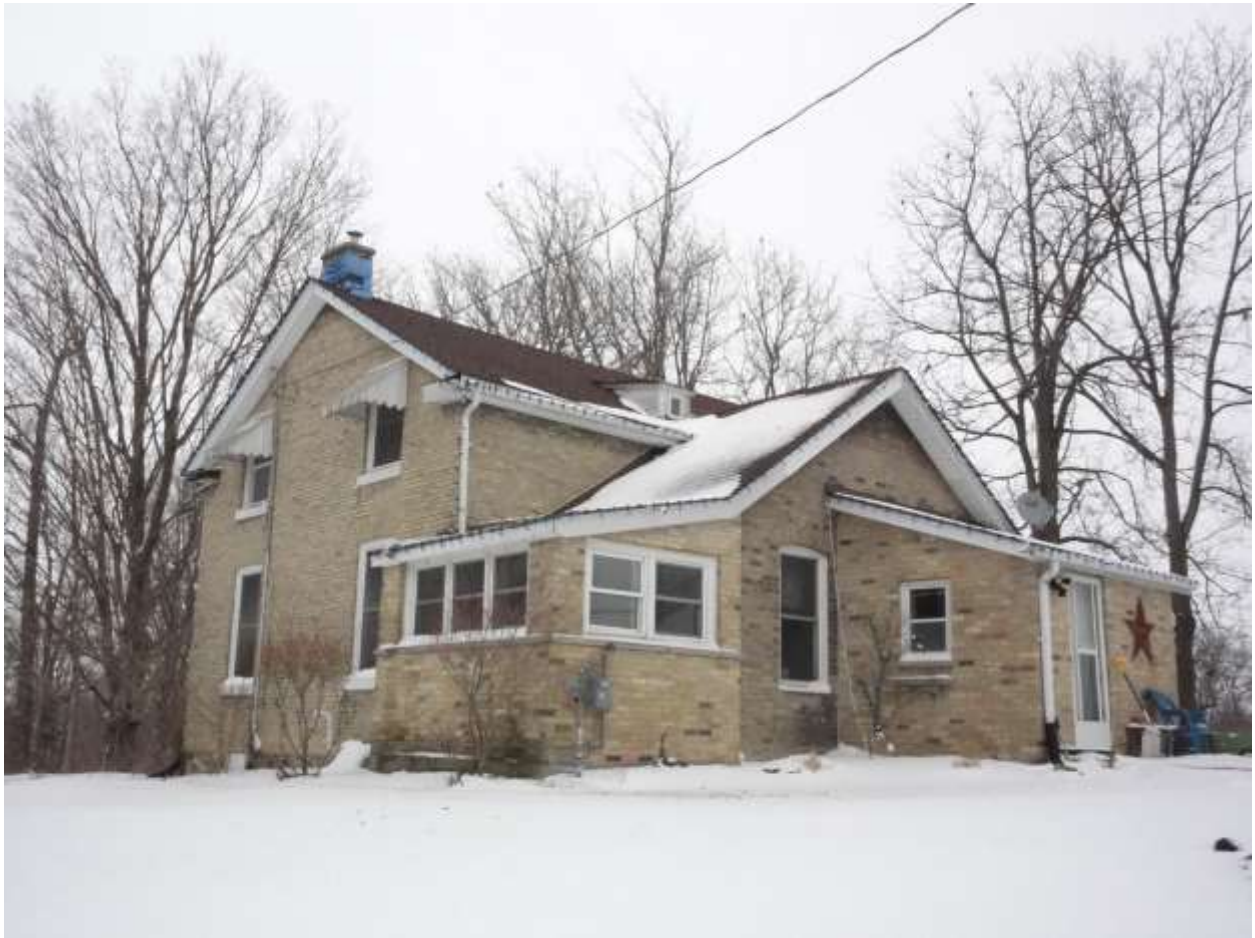
Image 13: Side elevation of house – west-south corner, with additions to original farmhouse (2019-02-14)
