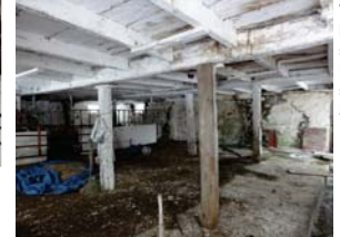
View of lower section of barn, stable area
