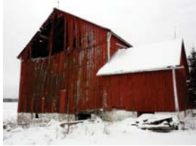
View of the barn and addition, east face
