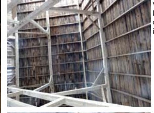
View looking up of barn interior
