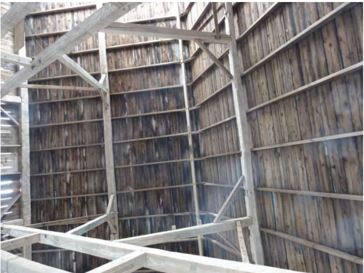
Image 8: View looking up of barn interior (2019-02-14).
