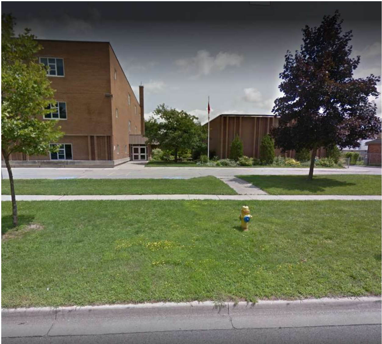
Image 2: Proposed location of proposed Pocket Park A, in front of 782 Waterloo Street (St. George's Public School) (courtesy Google, July 2018).
