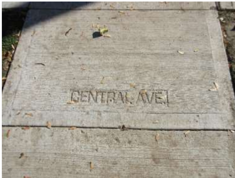
Image 16: Example of stamped street name in sidewalk concrete.
