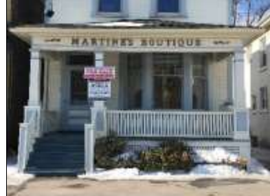
6. Porch, later addition
