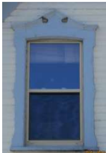
Image 6. Window Trim, 429 William Street, February 2019
