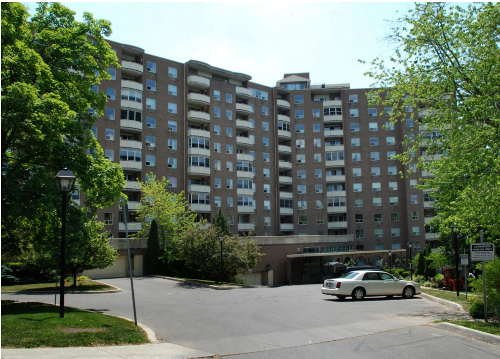
Figure 7 – 1 Grosvenor Street (Grosvenor Gates Apartment Complex)
