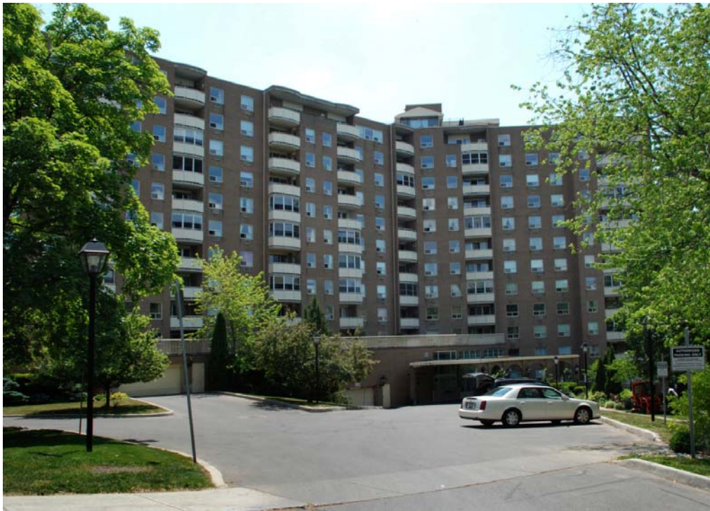
Figure 7 – 1 Grosvenor Street (Grosvenor Gates Apartment Complex)
