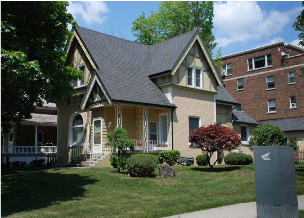
Figure 12 - 230 St. George Street
