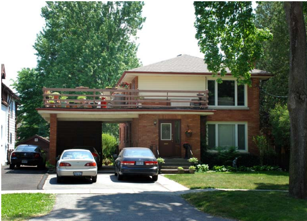
Figure 15 - 123 St. James Street
