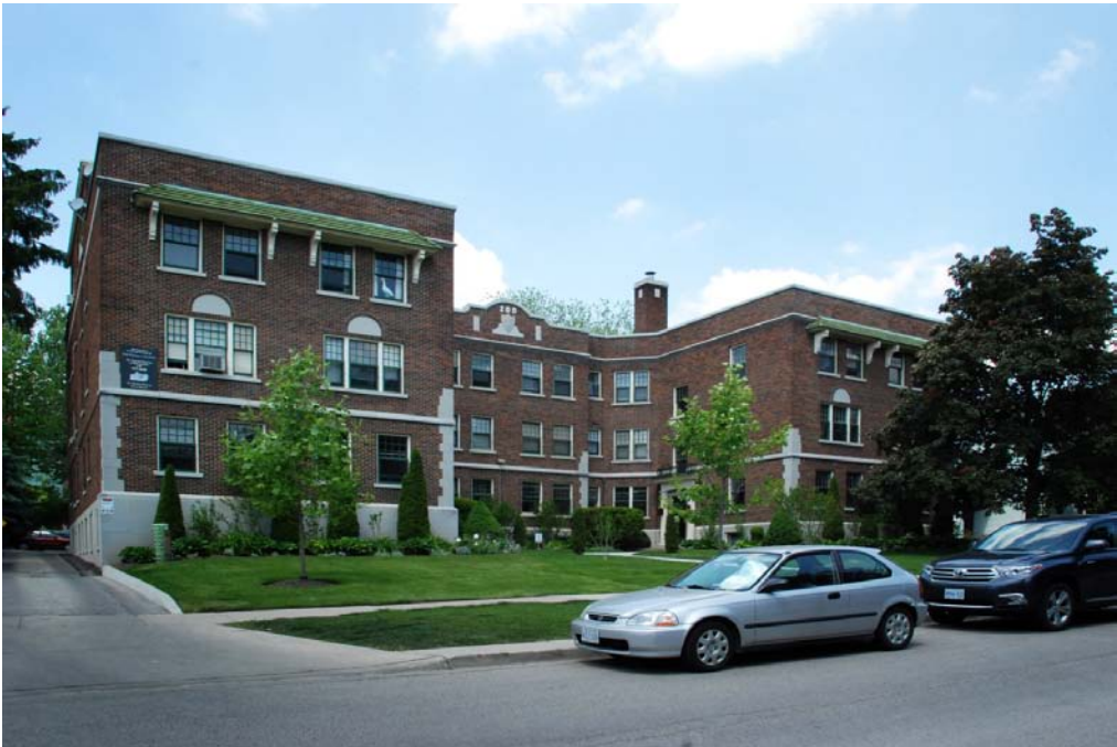
Figure 8 – 200 St. James Street
