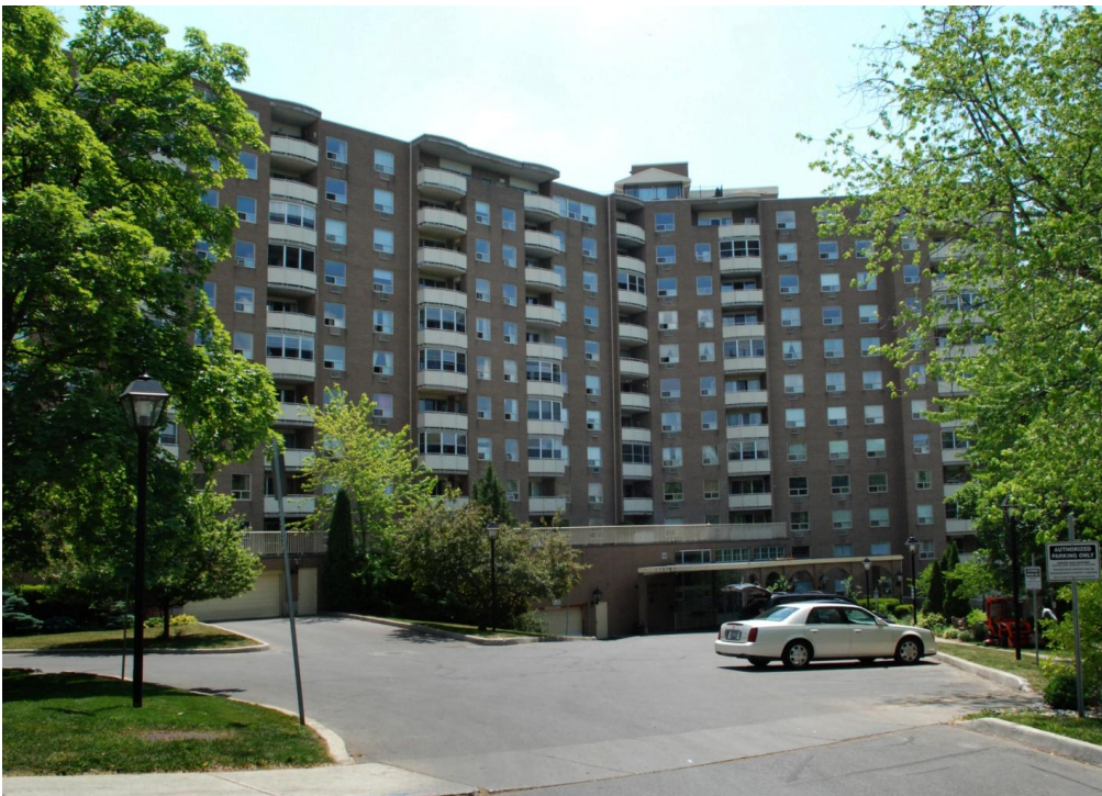
Figure 7 - 1 Grosvenor Street (Grosvenor Gates Apartment Complex)
