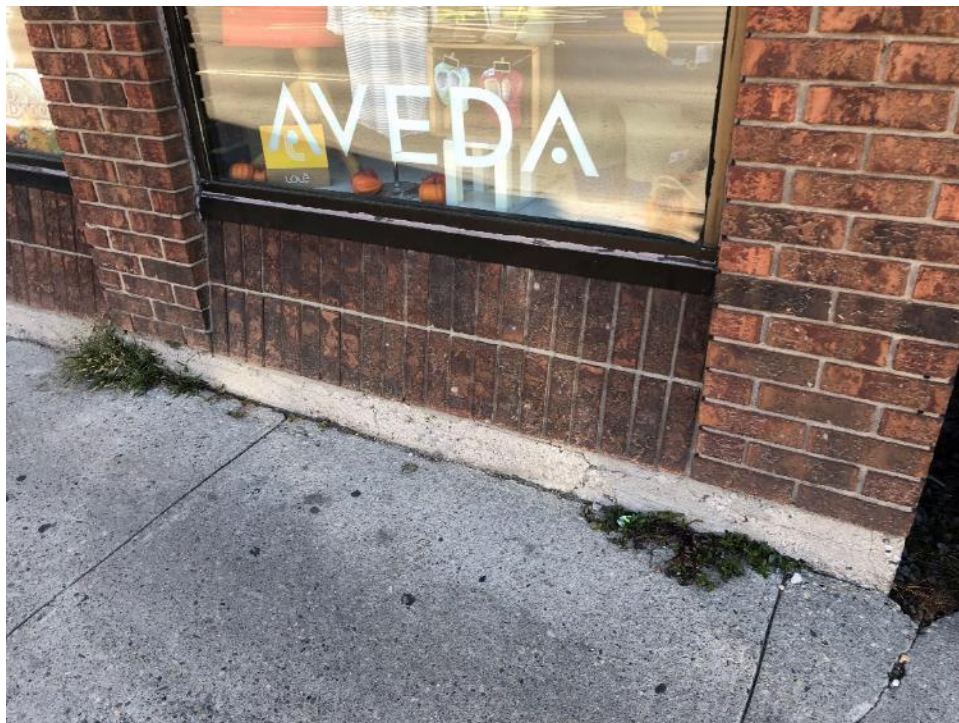
Image 18: Looking east at detail on front on front elevation of the building located at 740 Richmond Street, note the sloping brick. (WSP, 2018)
