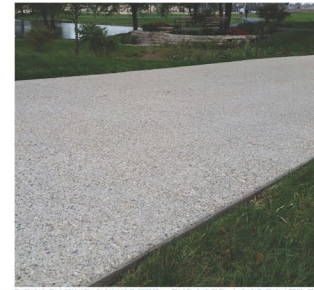
DECORATIVE CONCRETE - EXPOSED AGGREGATE FOR ACCENTS AND PATTERNING IN SPECIAL ZONES
