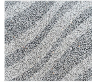
DECORATIVE CONCRETE - EXPOSED AGGREGATE FOR ACCENTS AND PATTERNING IN SPECIAL ZONES
