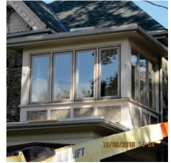
508 Waterloo Street after removal of the solarium windows
