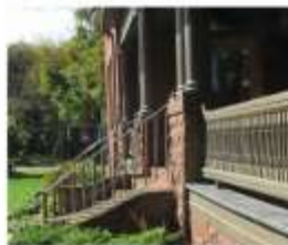
12. Porch: sandstone plinths, balustrade, columns, frieze, decking
