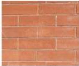
5. Red brick exterior cladding
