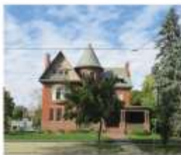
1. Form, scale, and massing of the building
