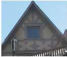
9. Half-timbering of the end-gables (north gable shown)
