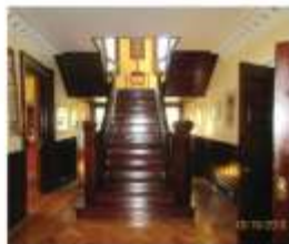
16. Wood, bifurcated main staircase (interior, first storey)
