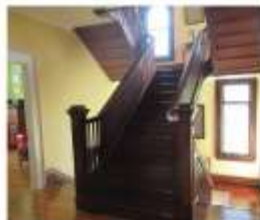
16. Wood, bifurcated main staircase (interior, second storey)
