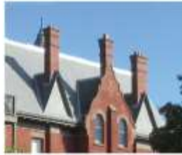
10. Four chimneys with decorative brick detailing (three shown)
