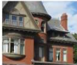
8. Hipped roof dormer with slight bellcast
