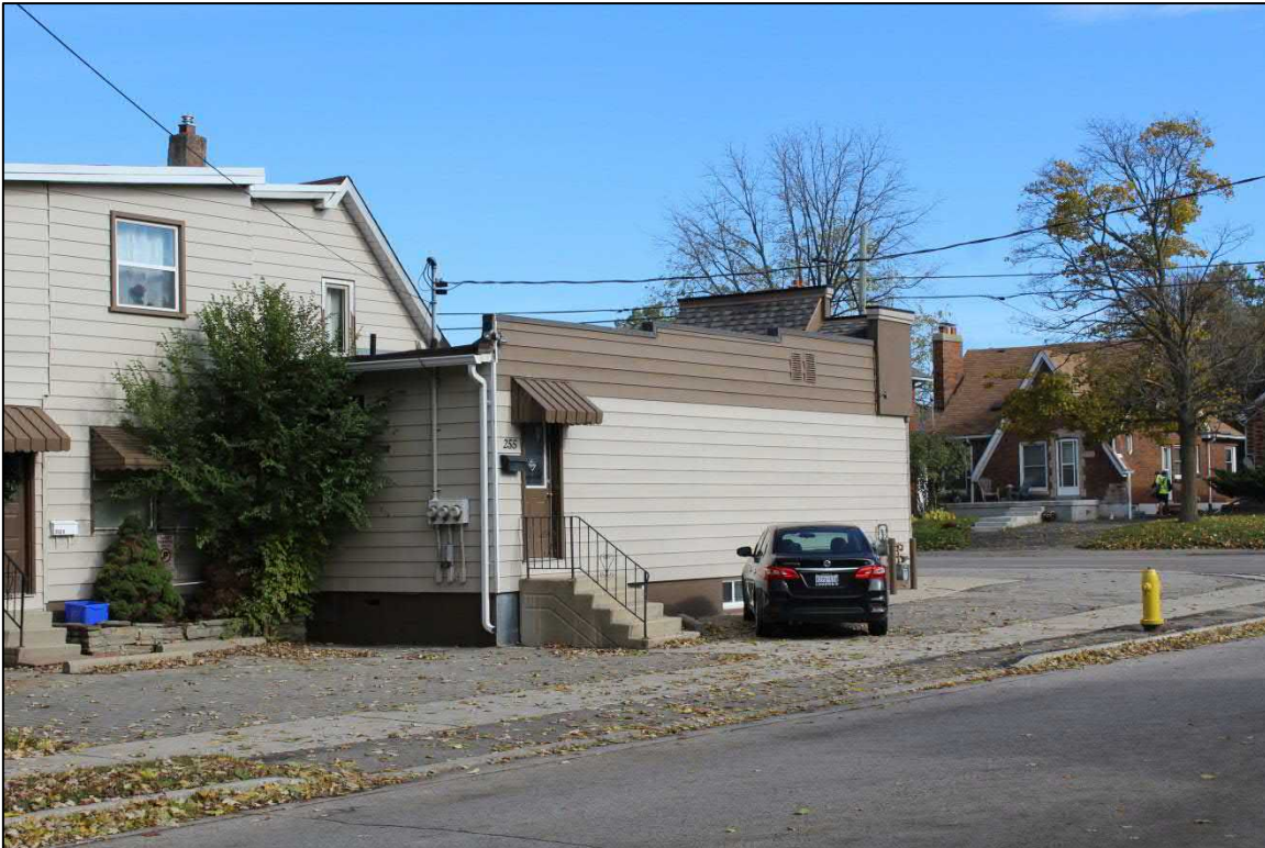
Image 5: Rear of storefront showing entrance door and boulevard parking. (AECOM, 2018)
