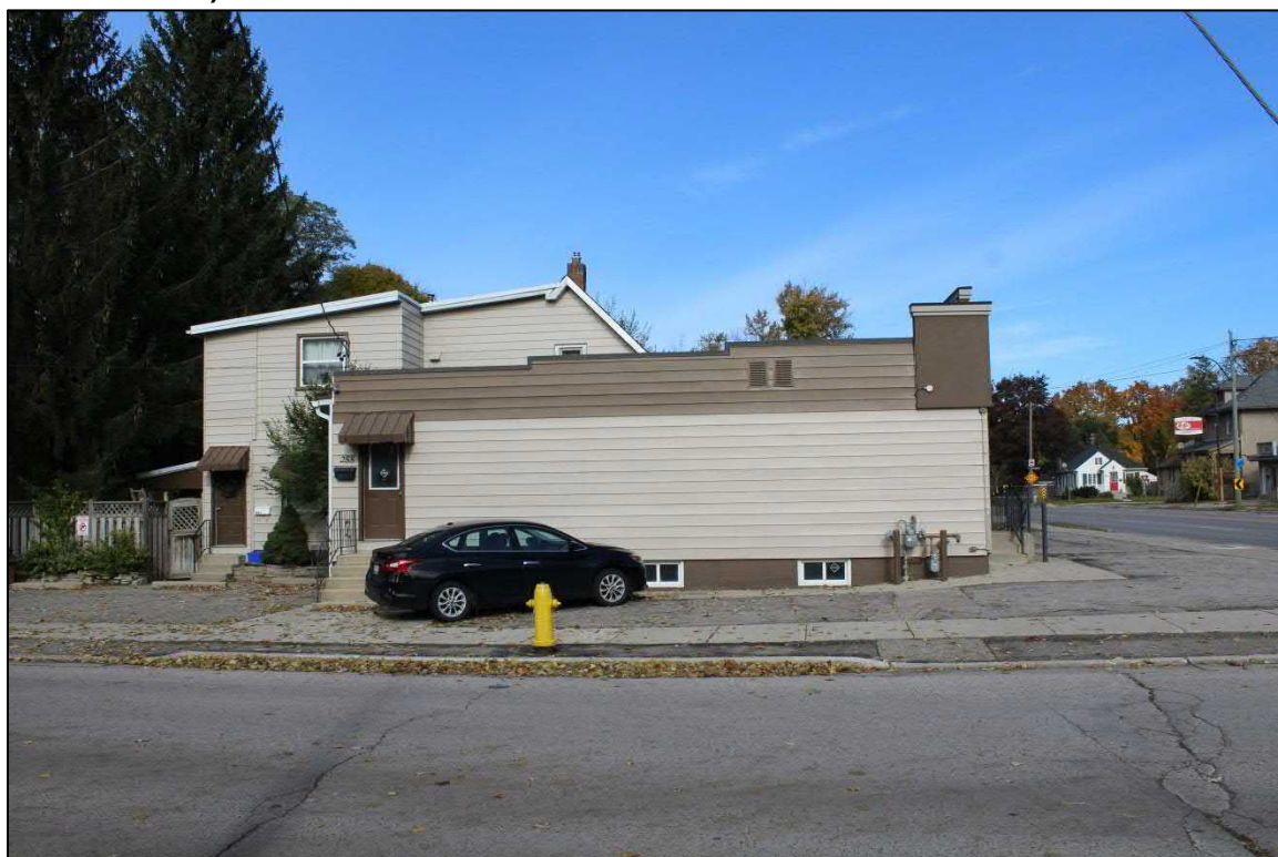
Image 4: South elevation, 255 Wellington Road; the two-storey residential unit at left appears to be a later addition. (AECOM, 2018)
