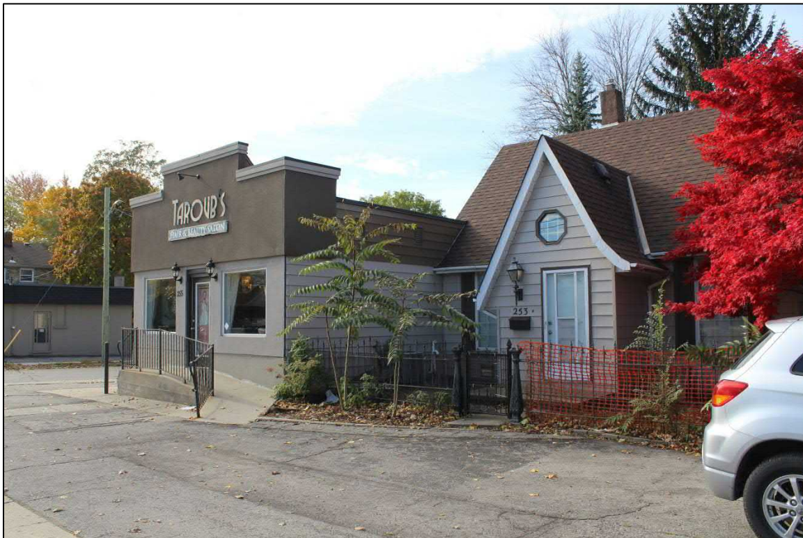
Image 3: Note the asymmetrical gable on the front of the house, and the wrought iron fence. The boomtown style front on the storefront is a recent addition. (AECOM, 2018)
