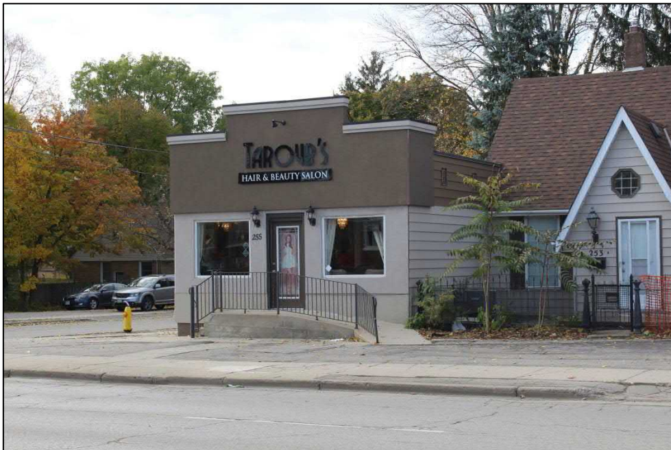
Image 2: Detail of storefront, 255 Wellington Road. (AECOM, 2018)
