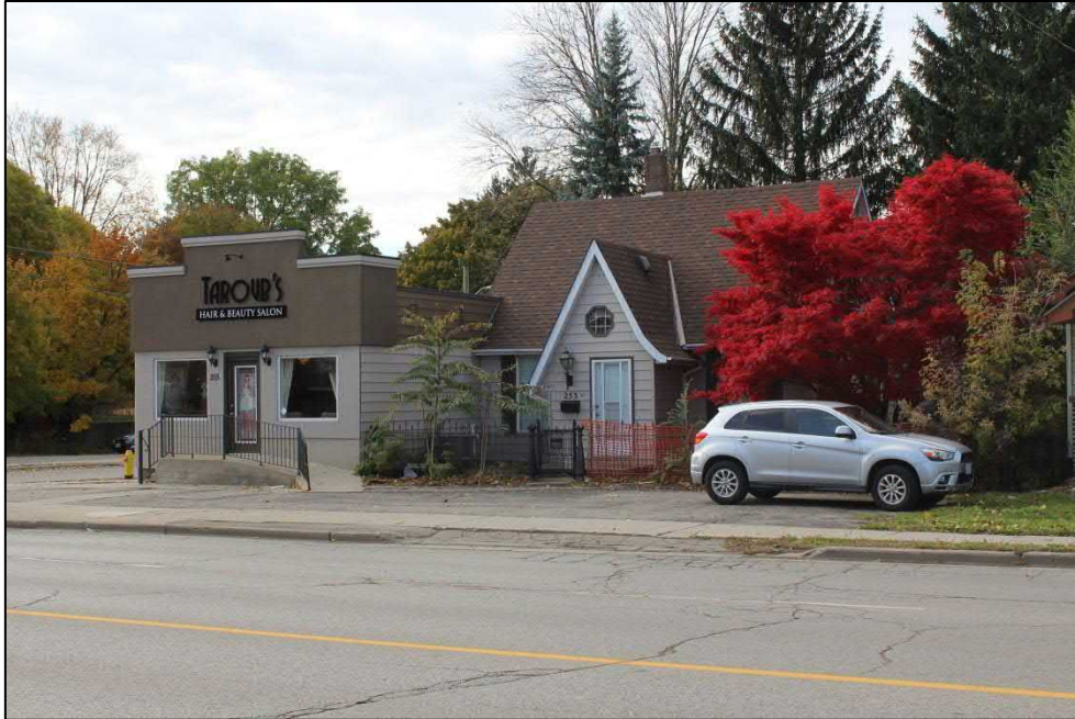
Image 1: 255 and 253 Wellington Road, showing commercial storefront at left with residential unit at right. (AECOM, 2018)
