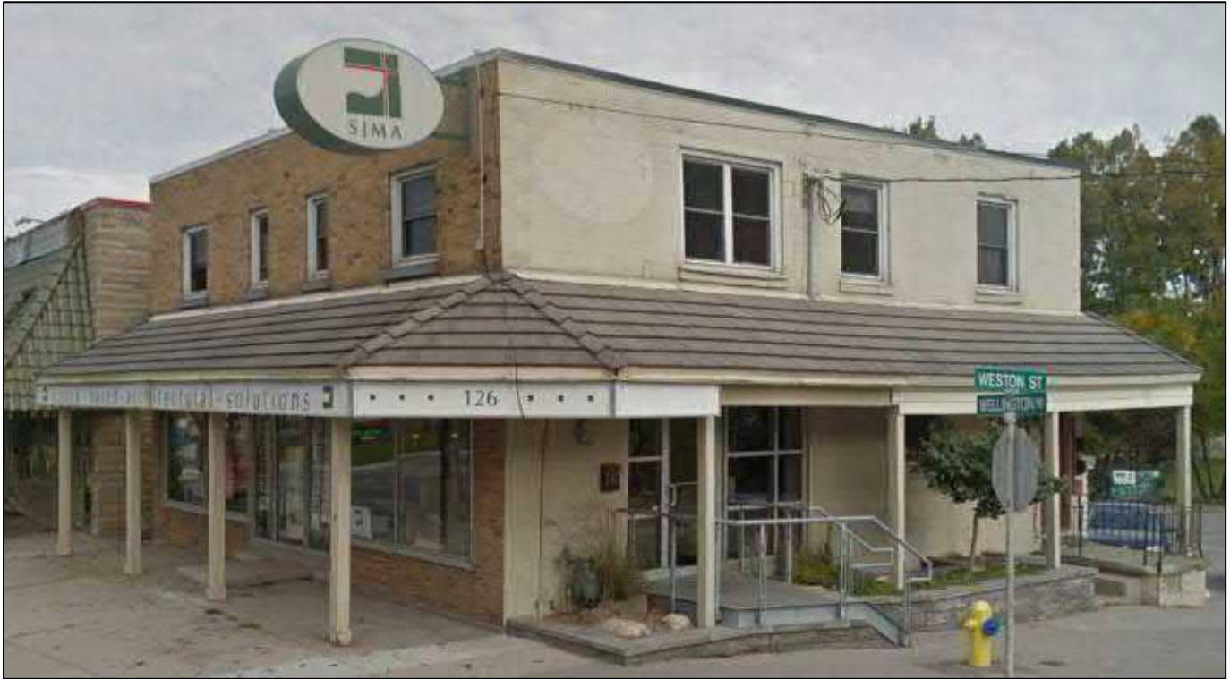
Image 7: View of building located at 126 Wellington Road, as shown from online street imagery showing exterior elevations and details prior to 2015 exterior alterations (2011)
