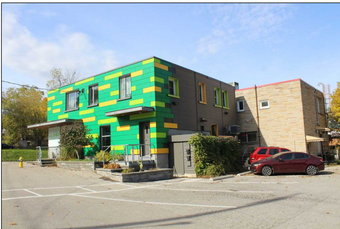
Image 6: South and east (rear) elevations of 126 Wellington Road, showing parking area and rear of 122 Wellington Road at right (AECOM, 2018).
