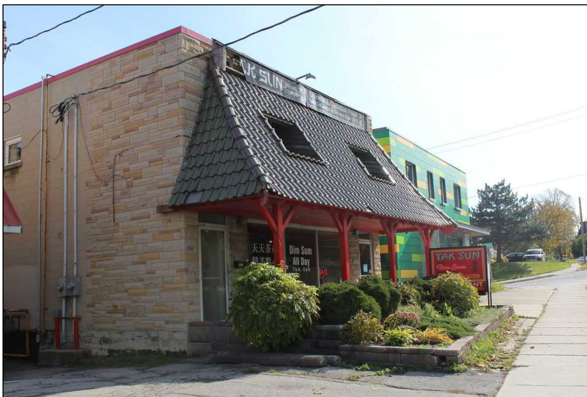
Image 3: 122 Wellington Road, showing portion of north elevation. (AECOM, 2018)
