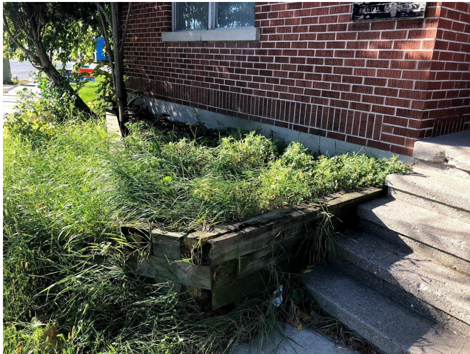
Image 10: View of the foundation and garden detail 44 Wharncliffe Road North.
