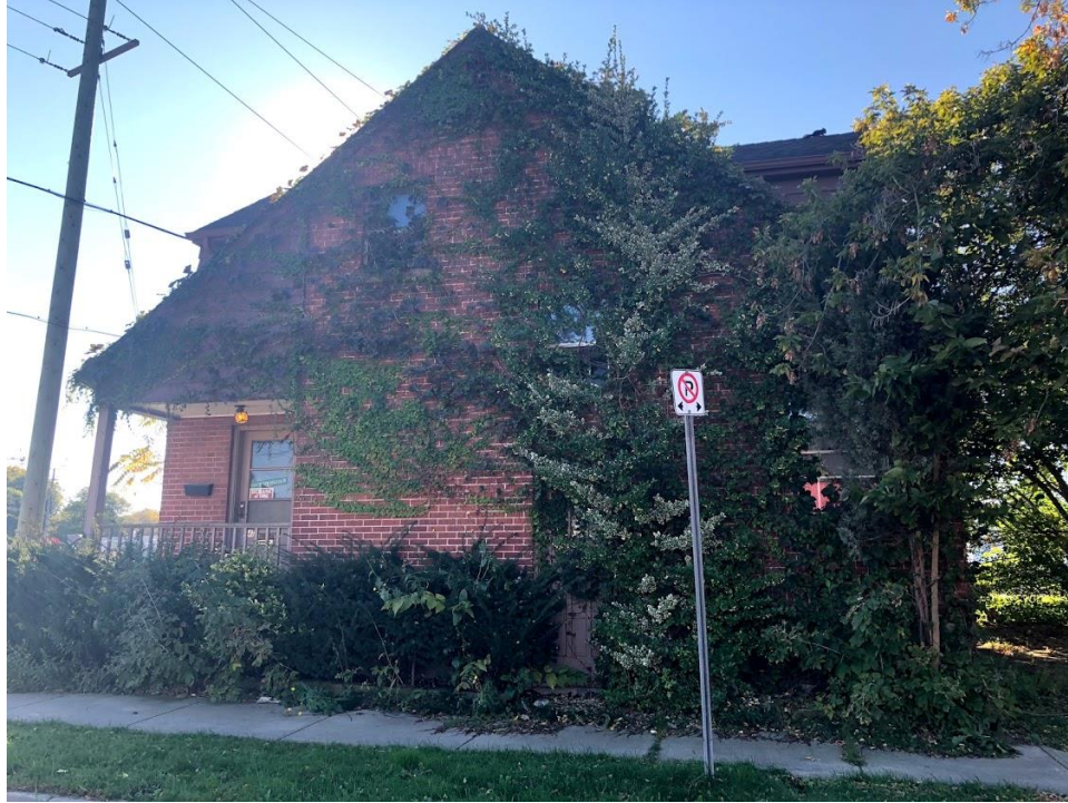
Image 3: View of the north side elevation of 44 Wharncliffe Road North, looking south.
