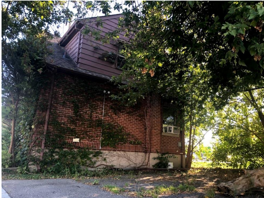
Image 6: View of the rear (west) elevation of 44 Wharncliffe Road North, looking southeast.
