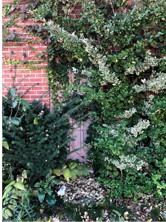
Image 9: View of the side entrance detail 44 Wharncliffe Road North.
