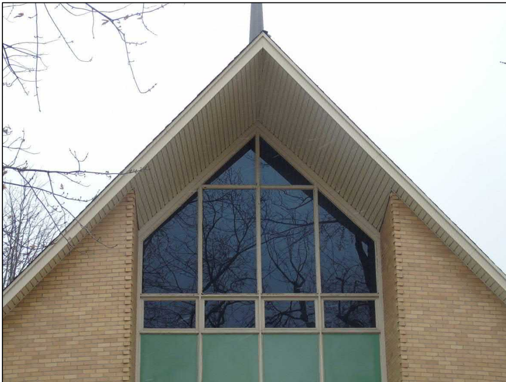
Image 12: Detail of windows and brickwork on east elevation of 1957 church. (AECOM, 2018)
