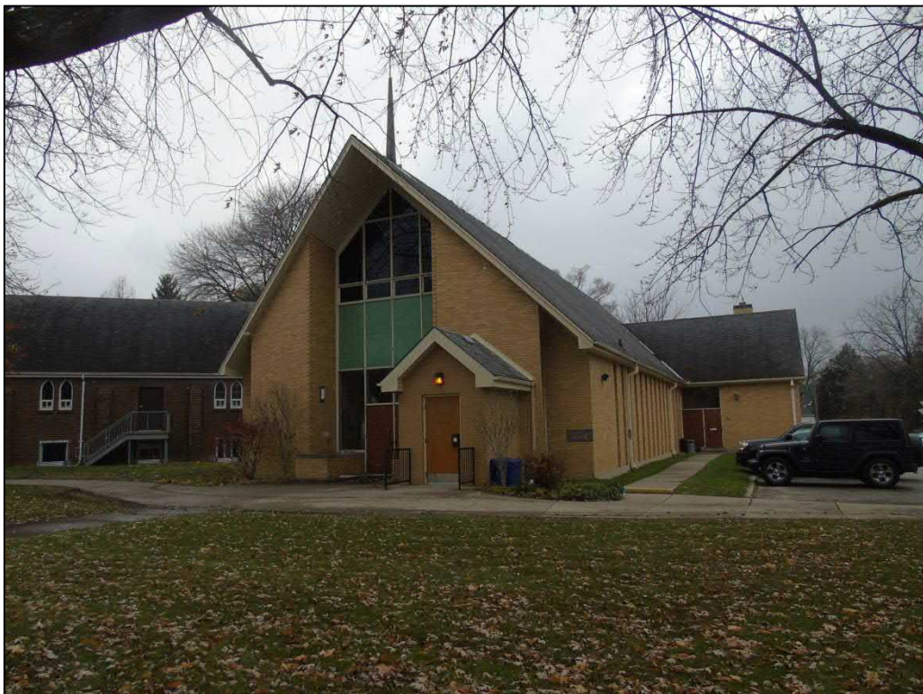
Image 8: 1957 church looking southwest from Wellington Road. (AECOM, 2018)
