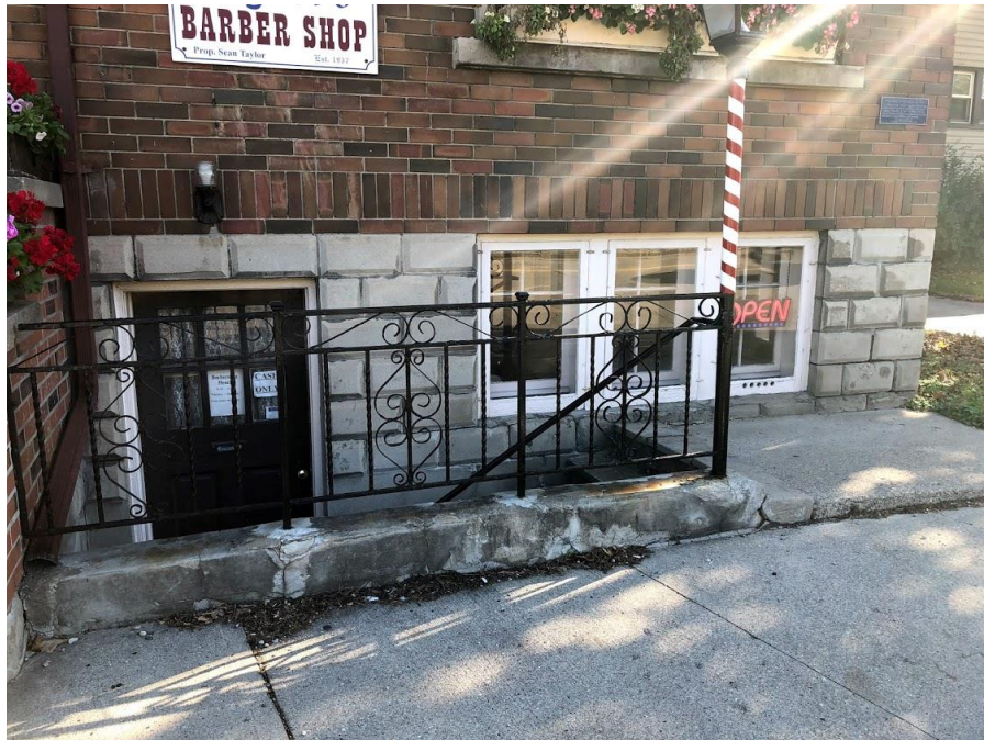
Image 5: View toward basement entrance on front elevation of the building located 1110 Richmond Street
