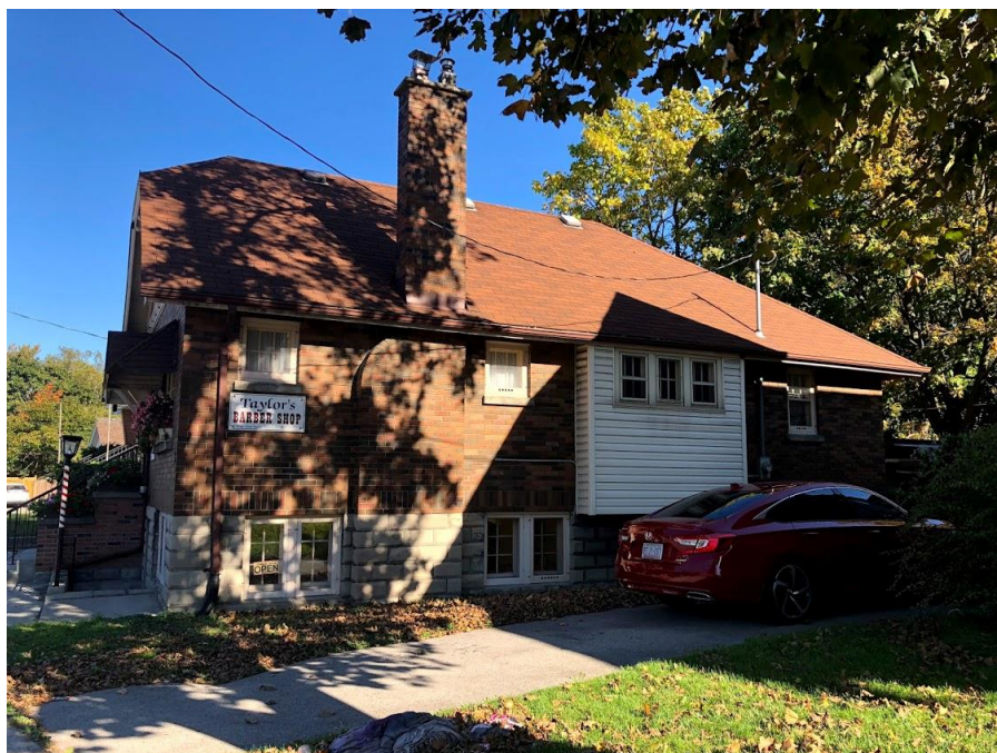
Image 12: View of south elevation including the curved detail of the chimney of the building located at 1110 Richmond Street
