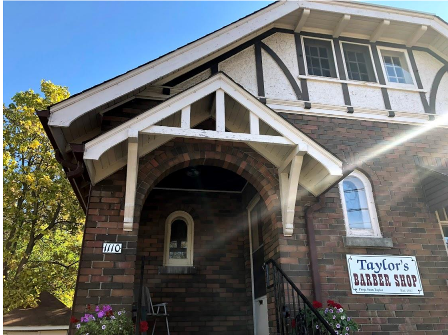
Image 7: View of front porch and gable awning on front elevation of the building located at 1110 Richmond Street
