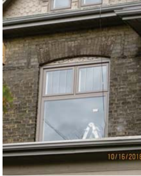
508 Waterloo Street after removal of the second floor main window
