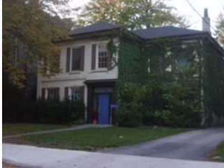
130 Kent Street. Owned by York Development ? Frat House. Listed on heritage inventory list.
