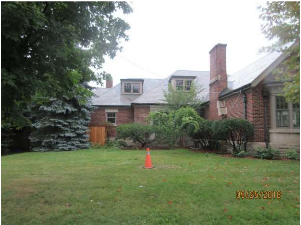
Image 4: Detail of the west façade of the existing built heritage resource located at 550 Dufferin Avenue. Note the profiles and fenestration of the windows located in the dormers.
