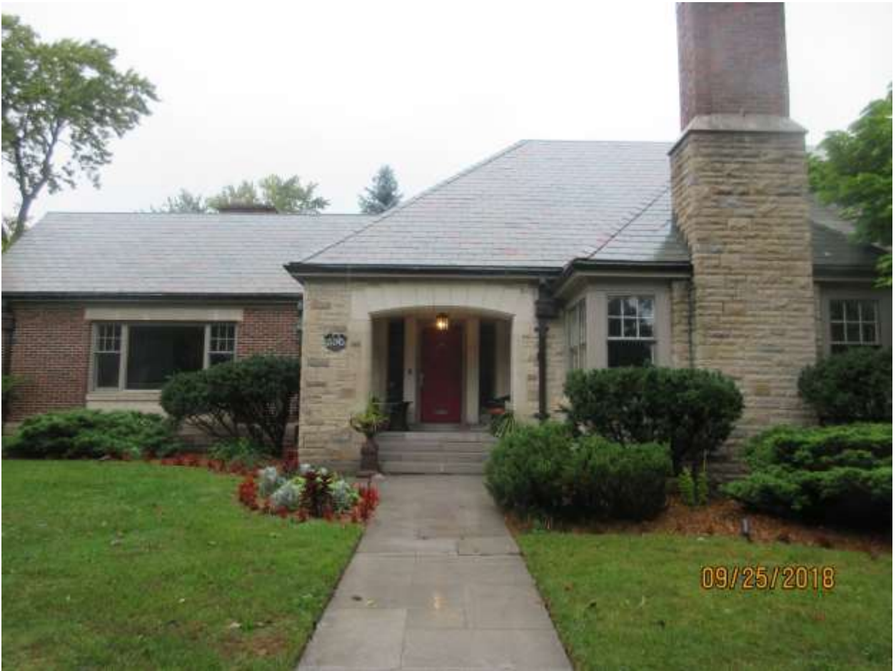
Image 2: Photograph of the main entry to the existing built heritage resource at 550 Dufferin Avenue.
