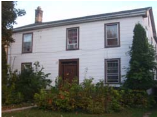
149 Central Ave. The house was built 1874. In the 1875 City Directory, Thomas Haskett, painter is living there. This property along with 155, 157 and 145 are being sold as one block for re-development for 2.2 million dollars. Listed on heritage inventory list.
