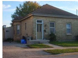
179 Ann Street ( recently purchased by York Development for re-development – next to old Carling Brewery site)
