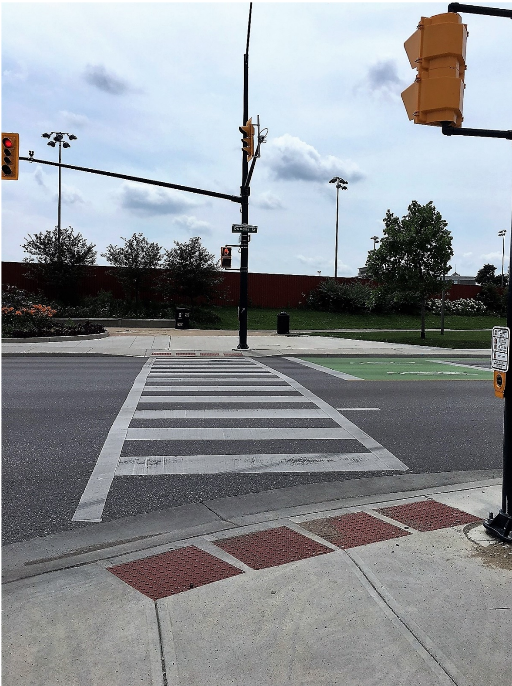
Accessible Pedestrian Control Signals and crosswalk at an intersection
