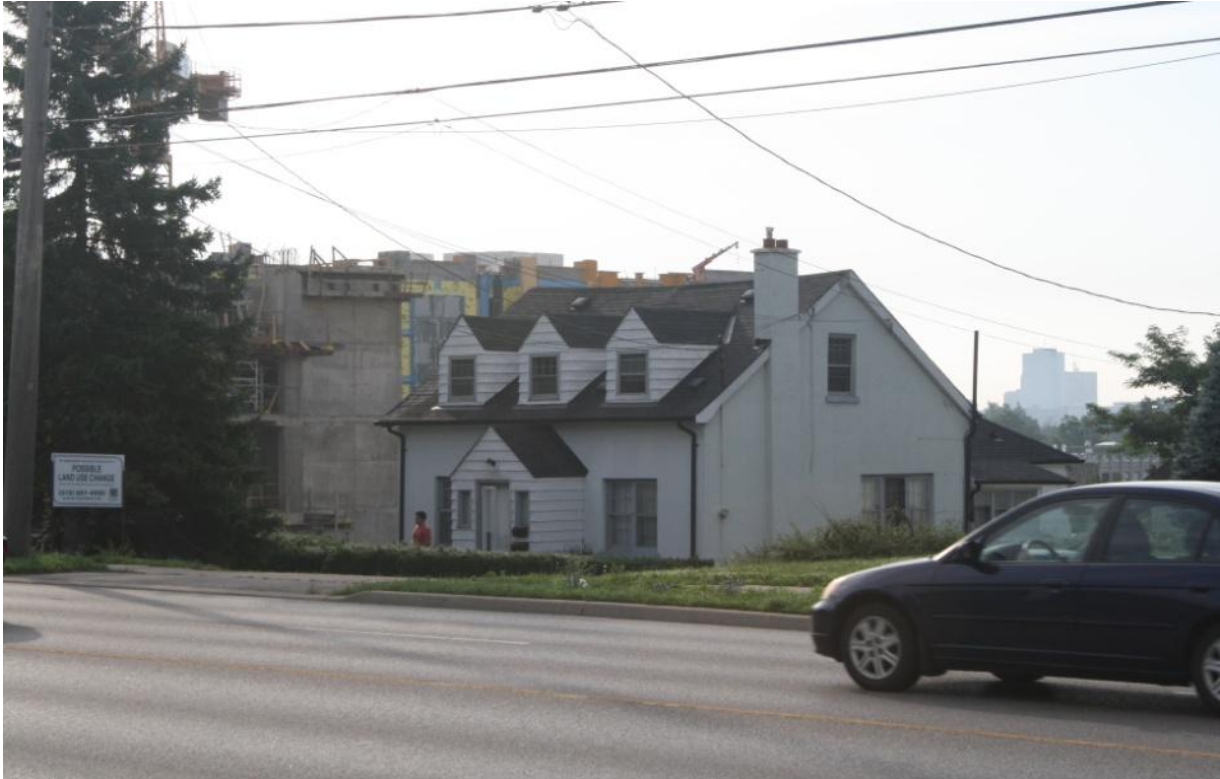
Construction East of Subject Site (underway)
