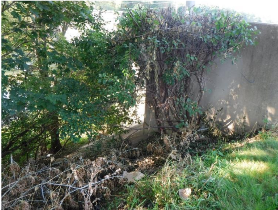
Plate 29: View of the northeast wingwall and steep slope of the embankment.
