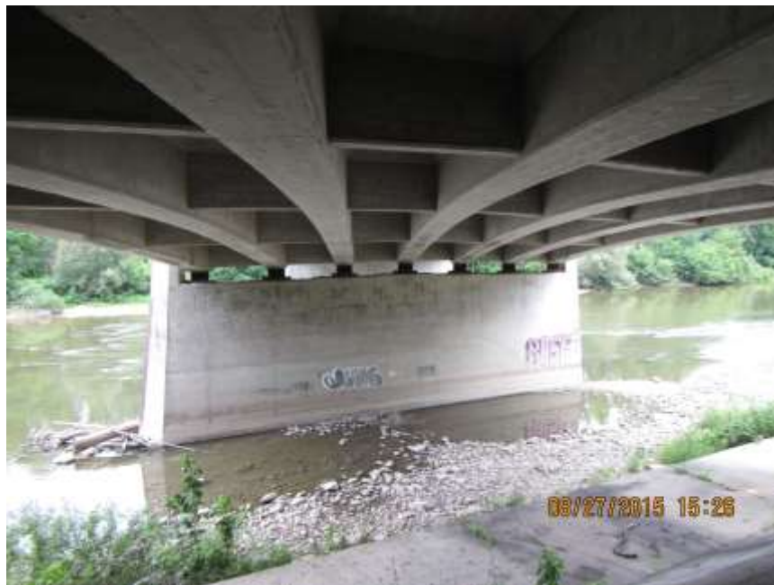
NORTH PIER - AUG'15
