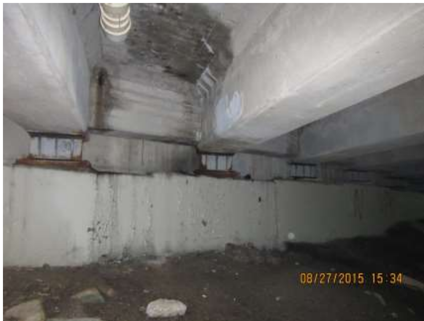
SOUTH ABUTMENT - AUG'15
