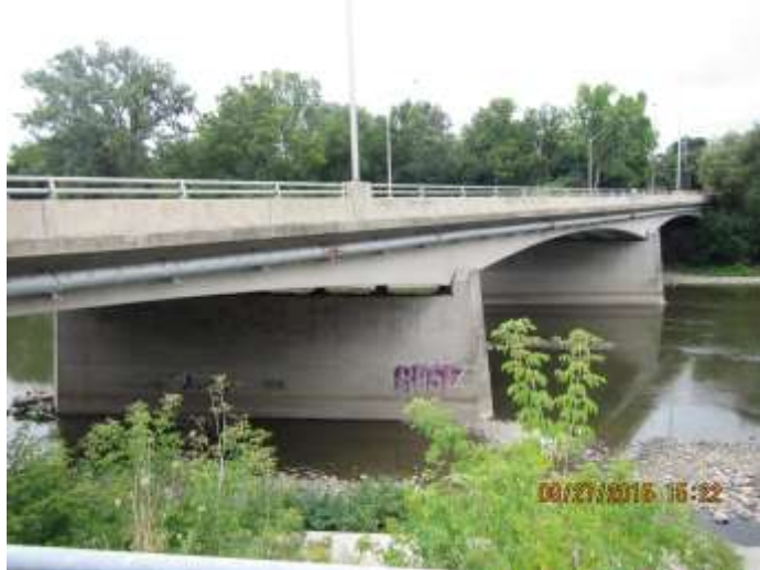
WEST ELEVATION LOOKING SOUTH - AUG'15
