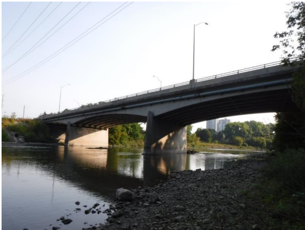
Plate 24: West elevation of bridge, view of watermain pipe.
