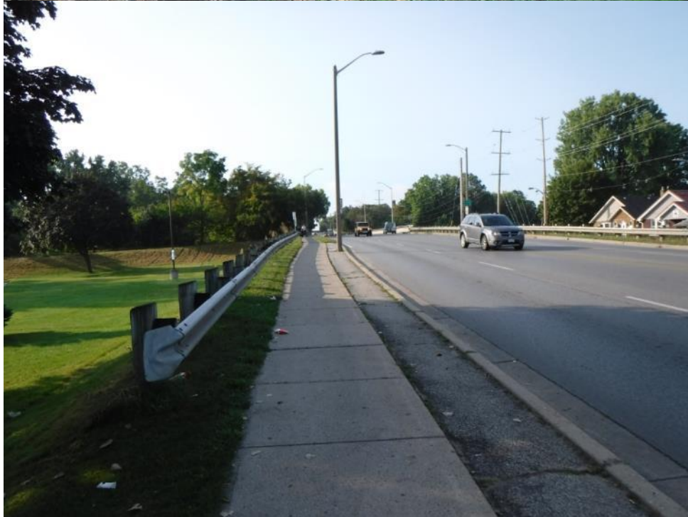
Plate 30: View of the north approach and the Blackfriars/Petersville HCD property to the left of the bridge.
