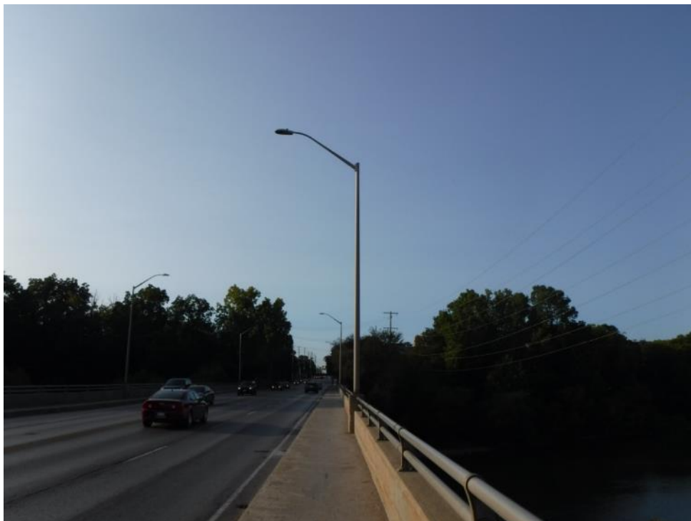
Plate 8: Pedestrian walkway on west side of bridge. View of the light standard.
