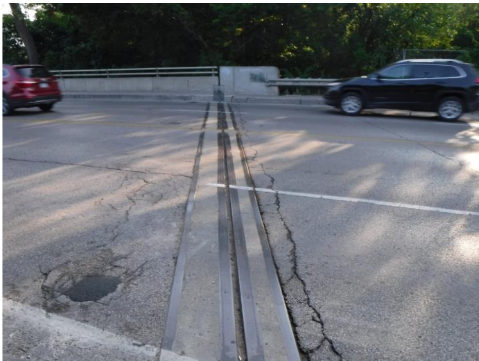
Plate 14: View of south expansion joint.
