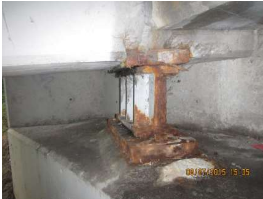
SOUTH ABUTMENT BEARING - AUG'15
