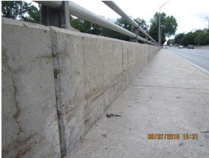
EAST PARAPET WALL - AUG'15
