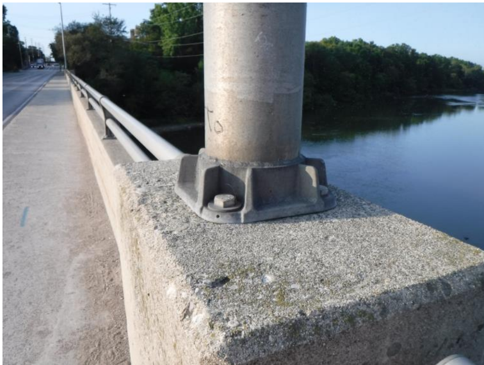
Plate 12: Base of light standard on the parapet post.
