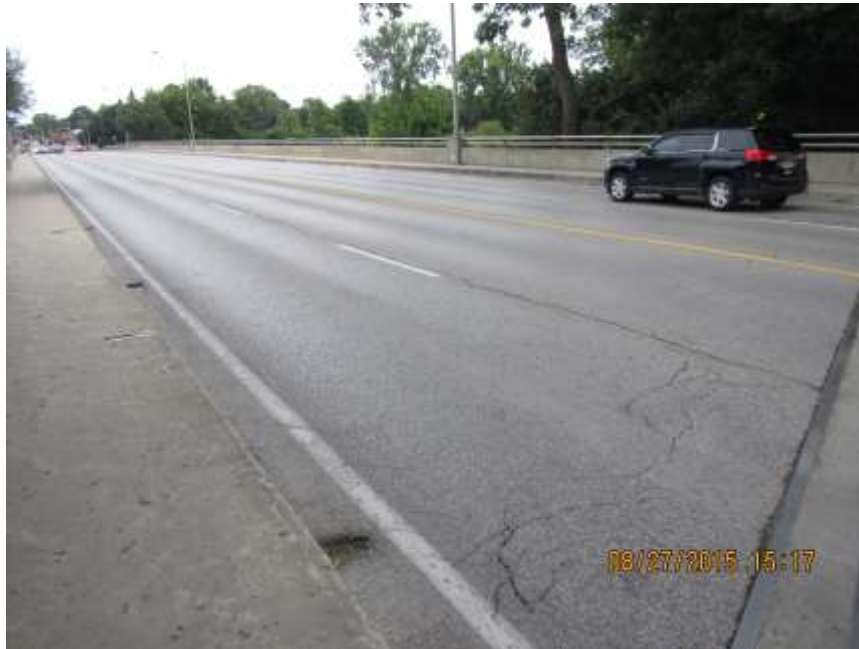
WEARING SURFACE LOOKING NORTH - AUG'15
