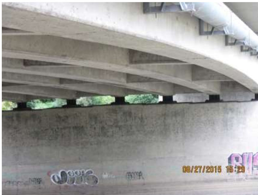
BEARINGS AT NORTH PIER - AUG'15
