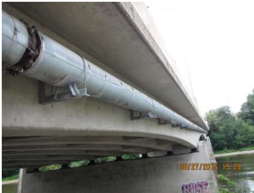
PIPE ALONG WEST SIDE OF BRIDGE - AUG'15
