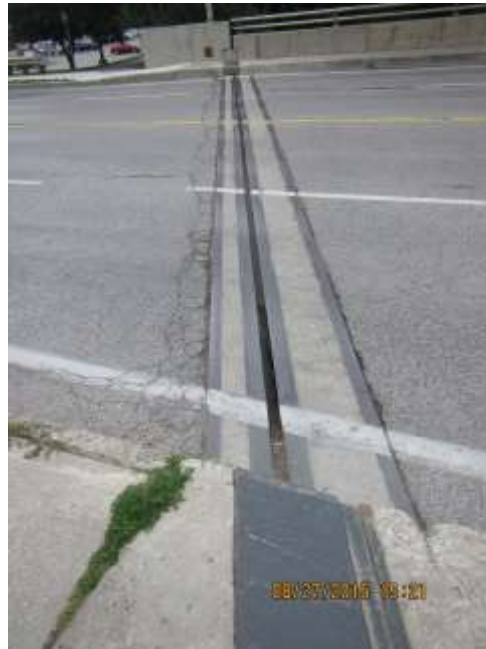
NORTH EXPANSION JOINT - AUG'15
