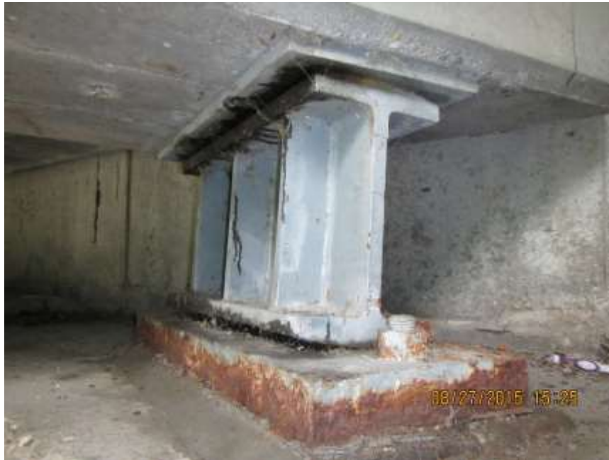
TYPICAL ROCKER BEARING - AUG'15
