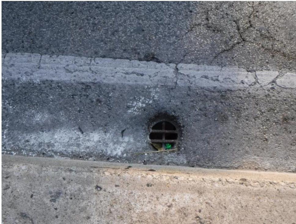
Plate 11: Example of the deck drains.
