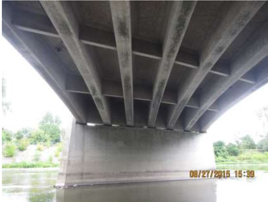
SECOND SPAN FROM THE SOUTH - AUG'15
