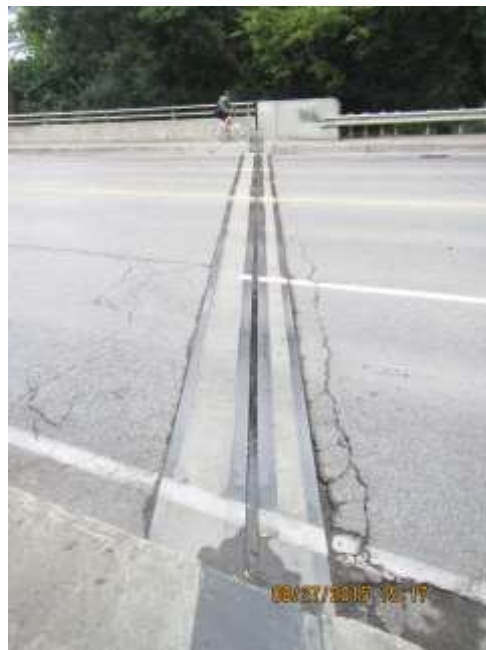
SOUTH EXPANSION JOINT - AUG'15
