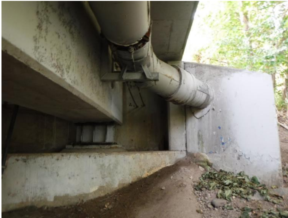
Plate 19: Close up of the south abutment.
