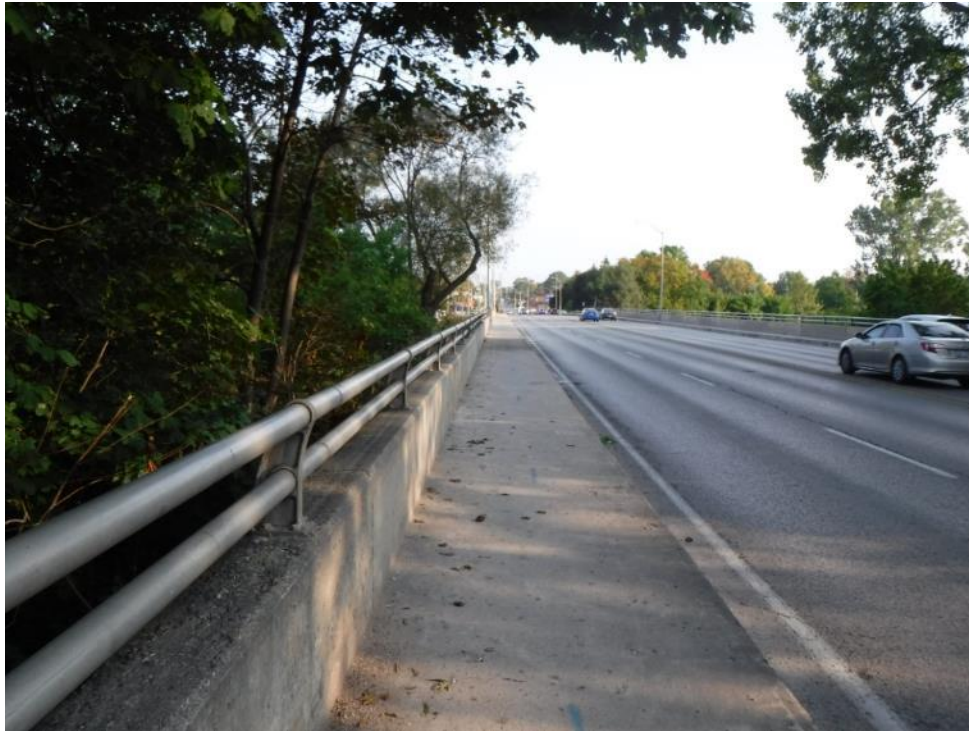
Plate 13: View of sidewalk, looking north.
