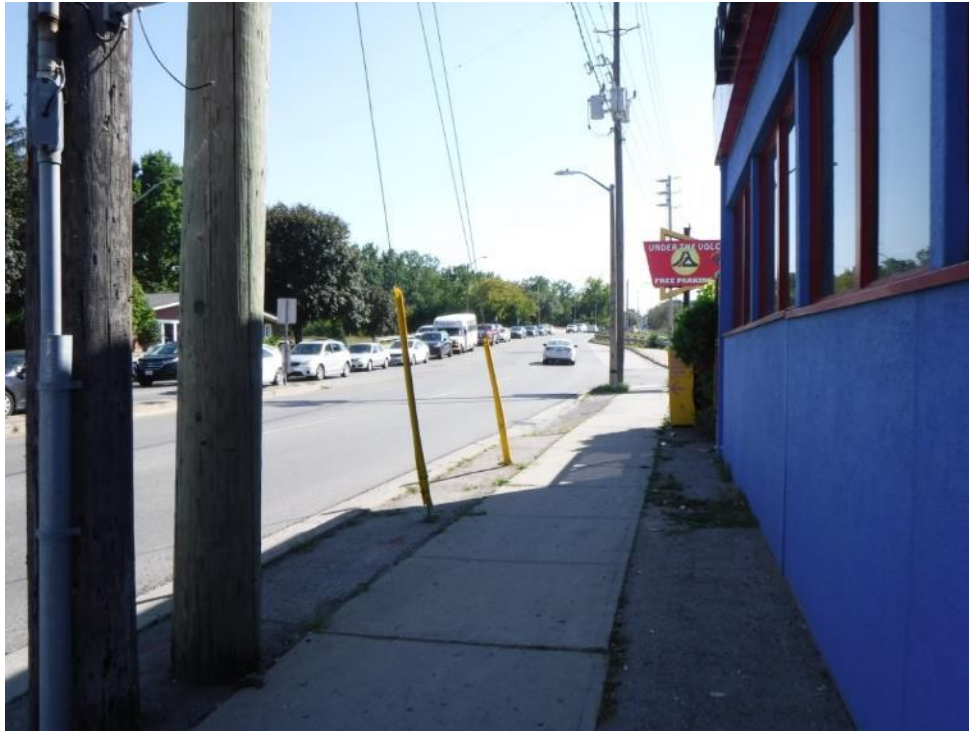
Plate 33: Looking towards the northern approach of the bridge from 30 Wharncliffe Road North.
