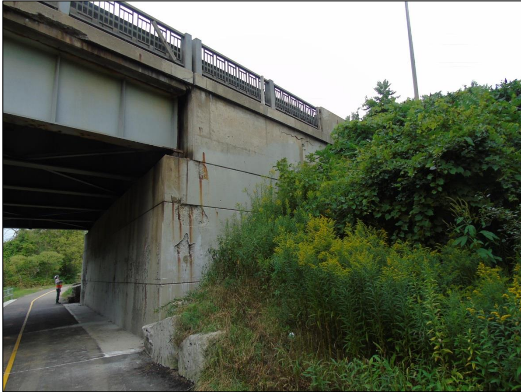
Photograph 14: View showing north abutment
