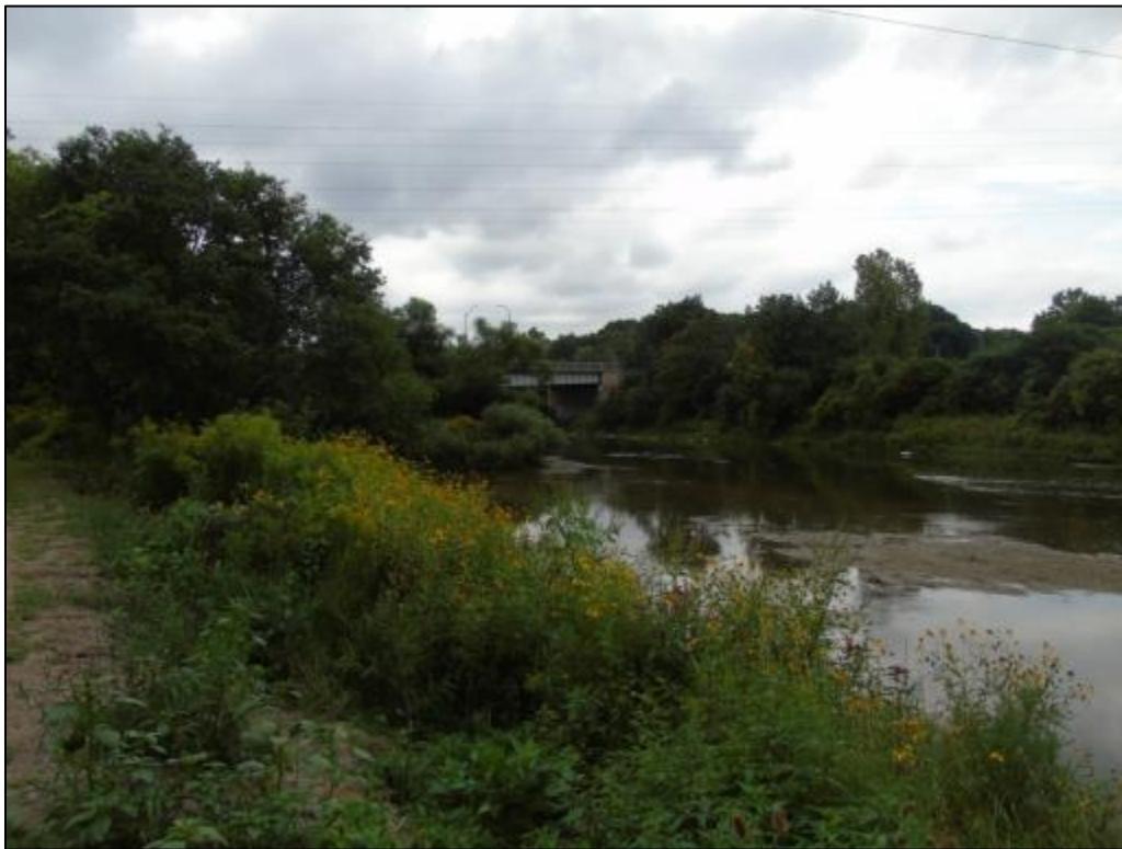
Photograph 1: View to Wenige Expressway Bridge in its setting over the South Branch of the Thames River
