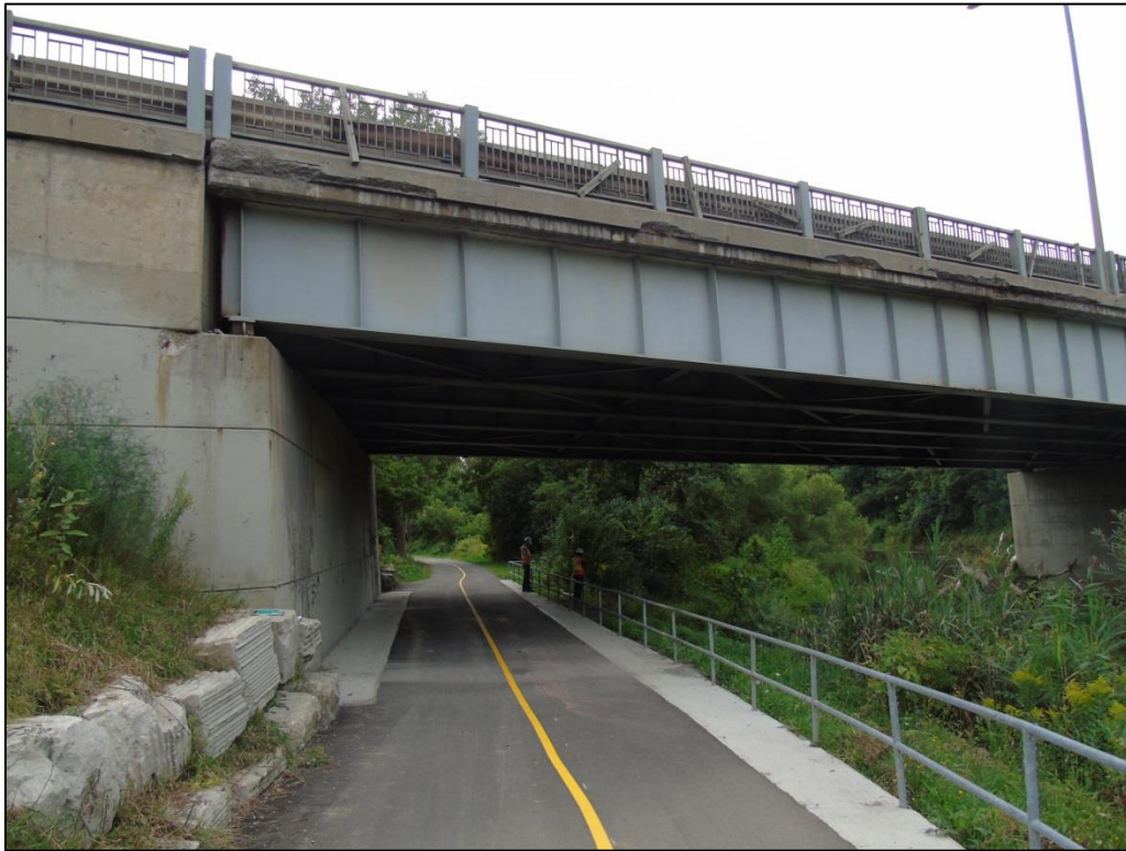
Photograph 10: View looking east towards bridge from Thames Valley Parkway
