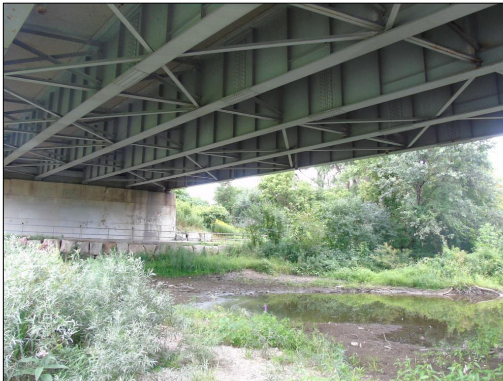
Photograph 19: View from pier showing welded steel plate girders
