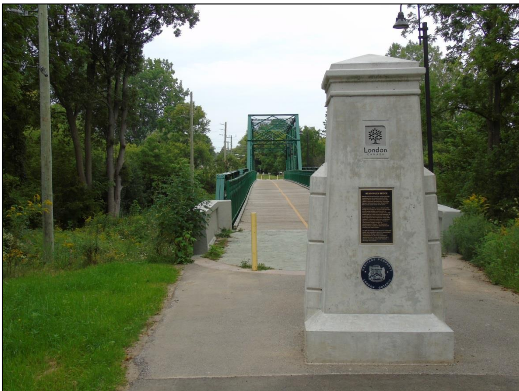
Photograph 7: Approach to Meadowlily Bridge, adjacent steel truss bridge located upstream
