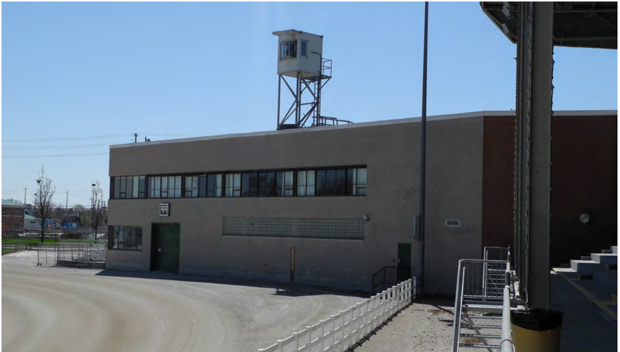
Figure 53 - The Carousel Room as seen from the Grandstand, provides considerable glazing to view the racetrack (CBCollective 2018).
