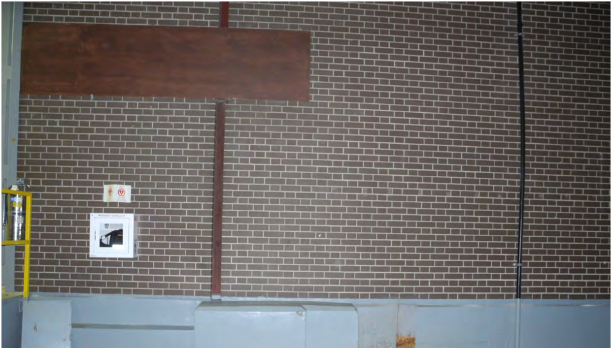
Figure 45 - The West Annex's east wall is the former exterior wall of the Progress Building (CBCollective 2018).
