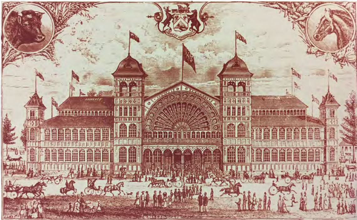
Figure 9 - Durand's Crystal Palace, though made of wood, eluded to Paxton's building with large amounts of glazing along with a prominent semi-circular central bay (Western Fair Archives as reproduced in Celebration of Excellence).
