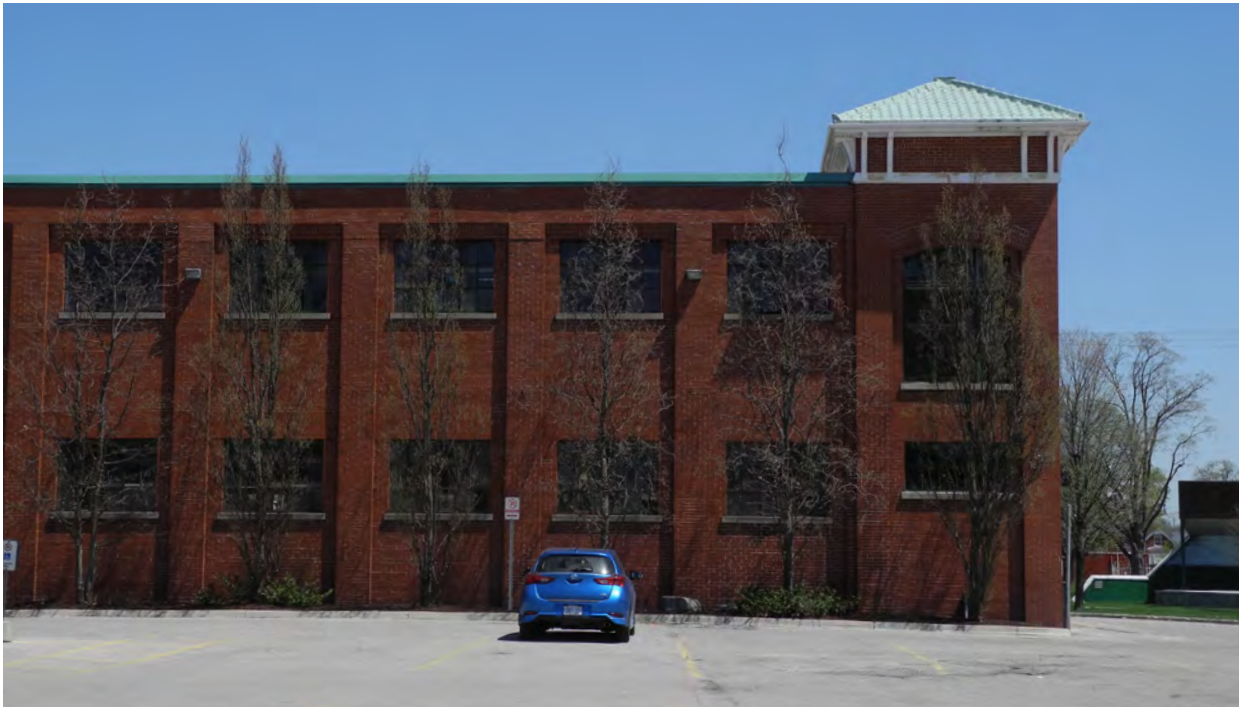
Figure 31 - The south end of the Confederation Building's west elevation, show recessed bays, steel sash windows, and elaborated corner towers (CBCollective 2018).
