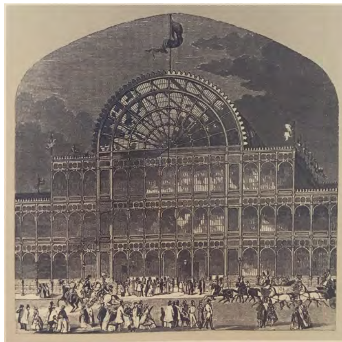
Figure 8 - Rendering of Paxton's 1851 Crystal Palace, with an incredible proportion of glazing on the building envelope, and a highly articulated structure (Western Fair Archives as reproduced in Celebration of Excellence).
