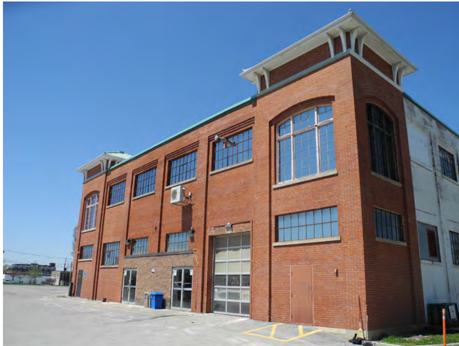
Figure 33 - South elevation of the Confederation Building, showing the differences in fenestration between the normal wall and tower windows (CBCollective 2018).
