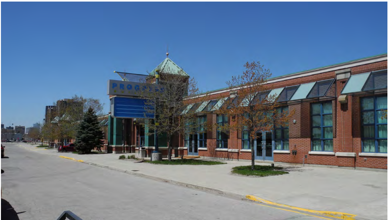
Figure 38 - The Progress Building (right), West Annex (centre), and Canada Building (left) all present as a single elevation, unified with post-modern detailing (CBCollective 2018).
