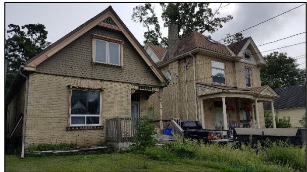
Figure 11: Example of housing in the surrounding area.
