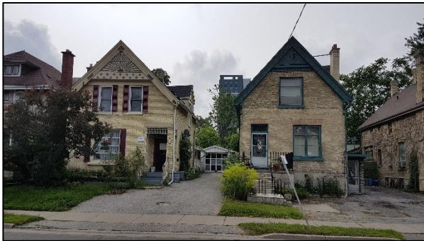
Figure 8: Example of housing in the surrounding area.
