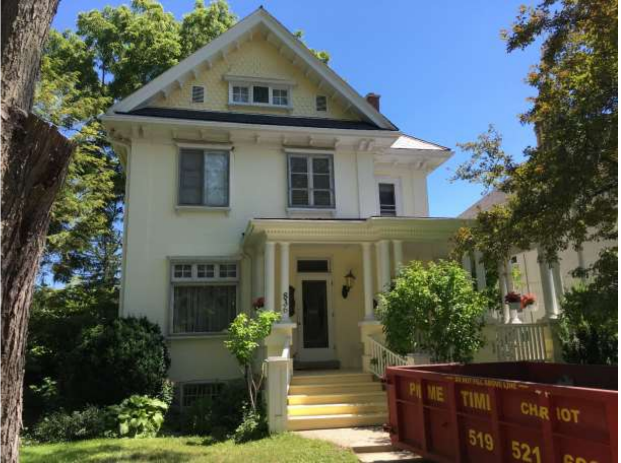
Image 3: View of the property located at 836 Wellington Street – during site visit on July 10, 2018
