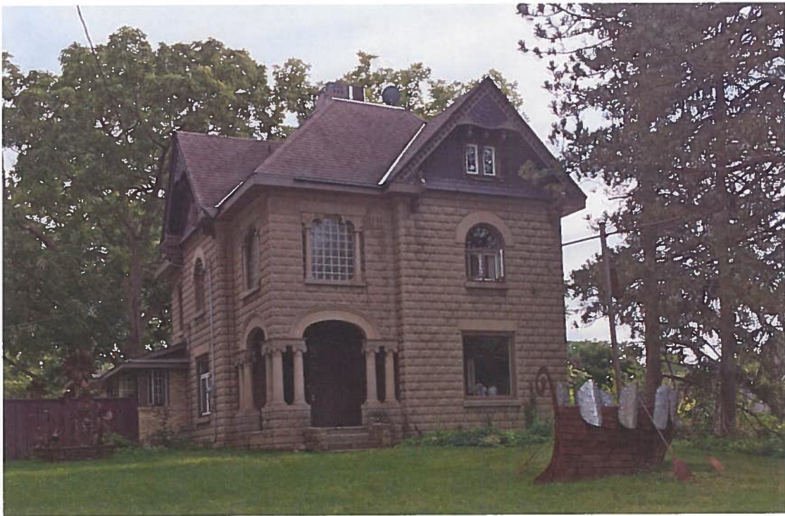
Heritage home to the immediate west of the proposed apartment structure
