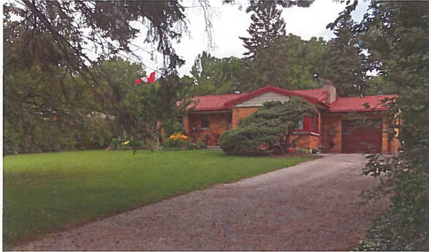
Single-storey house to the east of the proposed apartment structure
