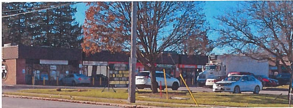
Single-storey plaza on the southwest corner
