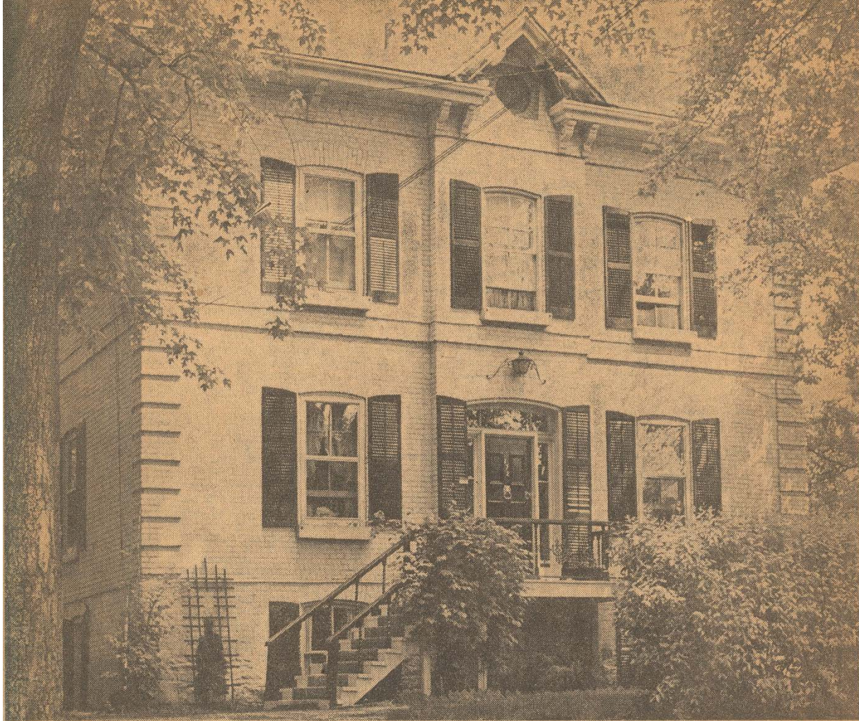
Image 1: Photograph of the property at 172 Central Avenue that was included in the London Free Press article "Escape March of Progress: Pioneer Homes Stand Firm" (June 30, 1962).
