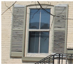
10. Wooden two-over-two wood windows
