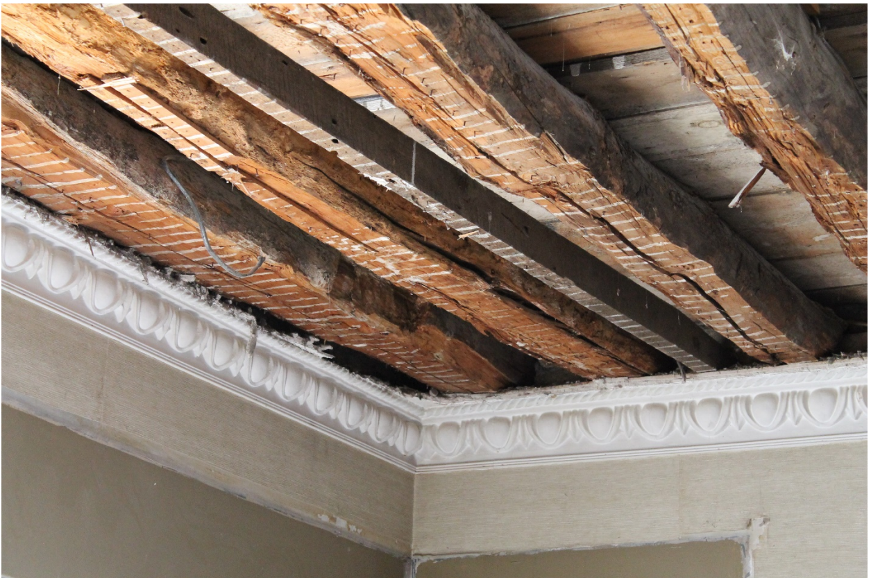
Image 8: Detail of the small portion of the egg-and-dart plaster moulding which remains on the interior of the building located at 172 Central Avenue (May 1, 2018).
