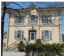
5. Symmetrical, three-bay facade with middle bay slightly projecting
