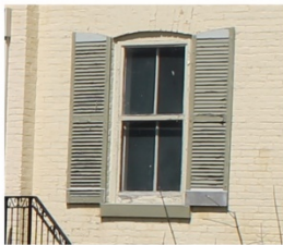
9. Segmented arch window openings with radiating brick voussoirs
