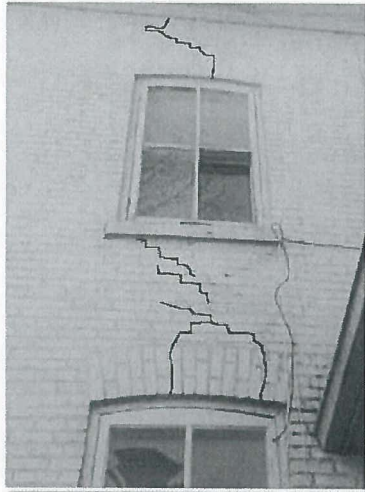
Image 5: Rear Brick Wall
