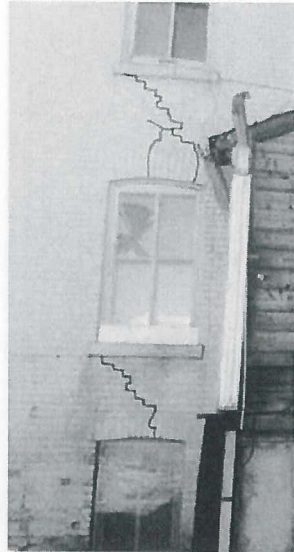
Image 6: Rear Brick Wall
