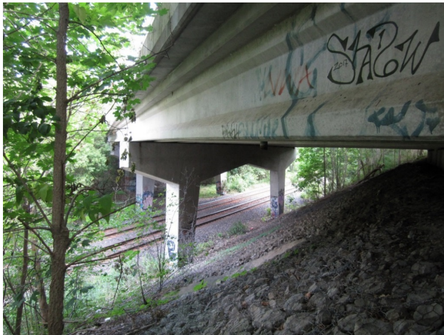
Plate 11: View looking northeast beneath the bridge towards the cast in place concrete piers
