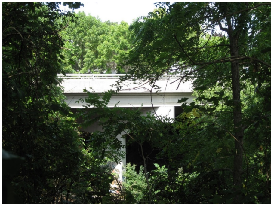
Plate 9: View looking north of the Riverside Bridge through vegetated area south of the bridge
