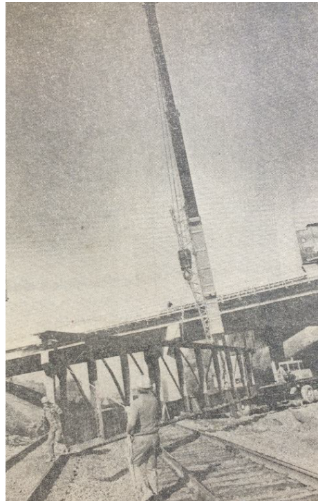
Plate 3: Construction crews remove the steelwork of the old Riverside Bridge, October 1974 (London Free Press, October 9, 1974)
