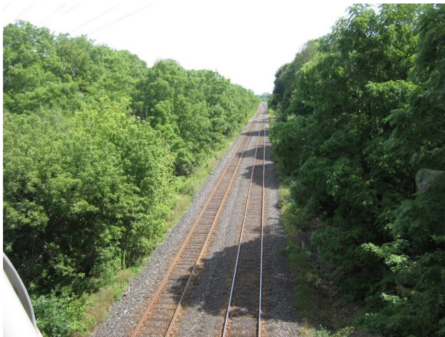
Plate 7: View of railway tracks looking south
