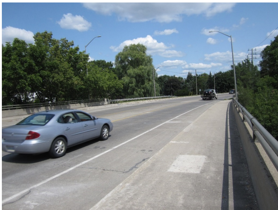
Plate 12: View looking northeast across the Riverside Bridge
