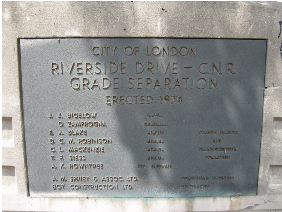
Plate 16: Detail view of the plaque at the northeast end post of the bridge
