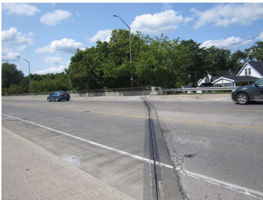
Plate 14: View looking northwest at the expansion joint of the Riverside Bridge
